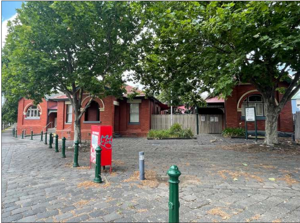
Figure 12 The north elevation of the former Saleyard's administration building.
