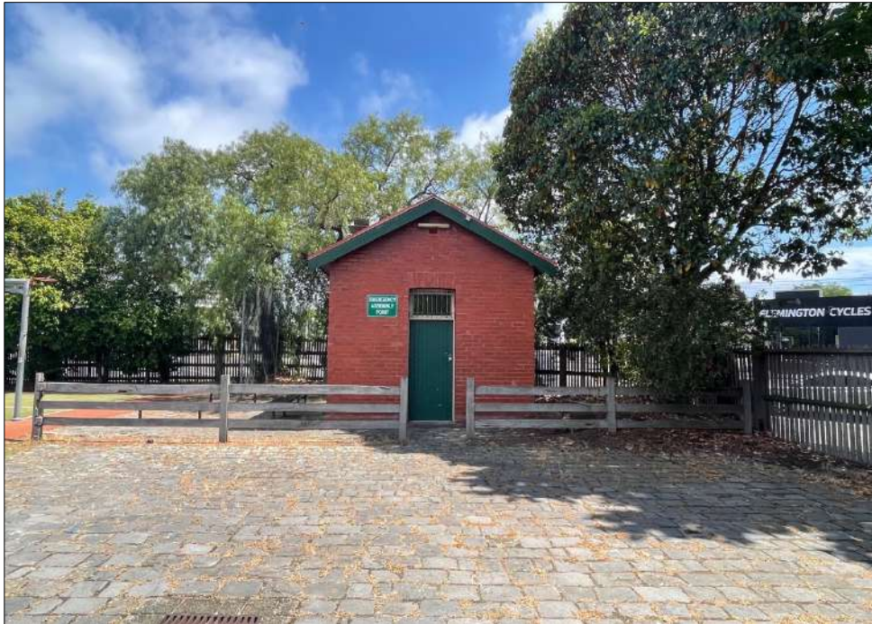
Figure 8 View looking north towards the Drover's Hut.
