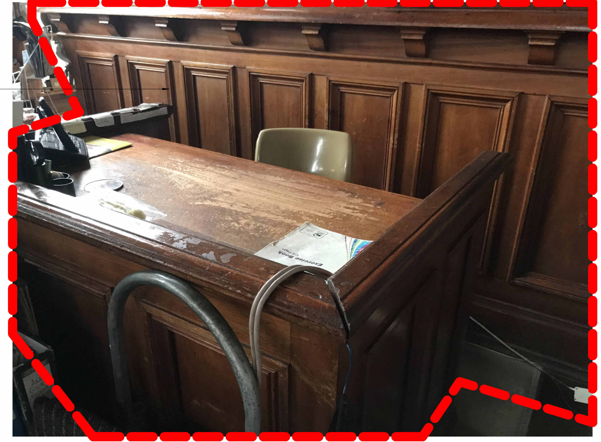
Restore existing Judge desk and clerks desk, removed existing vinyl flooring and make good as require. light sand and re-oil to match existing colour tone.
