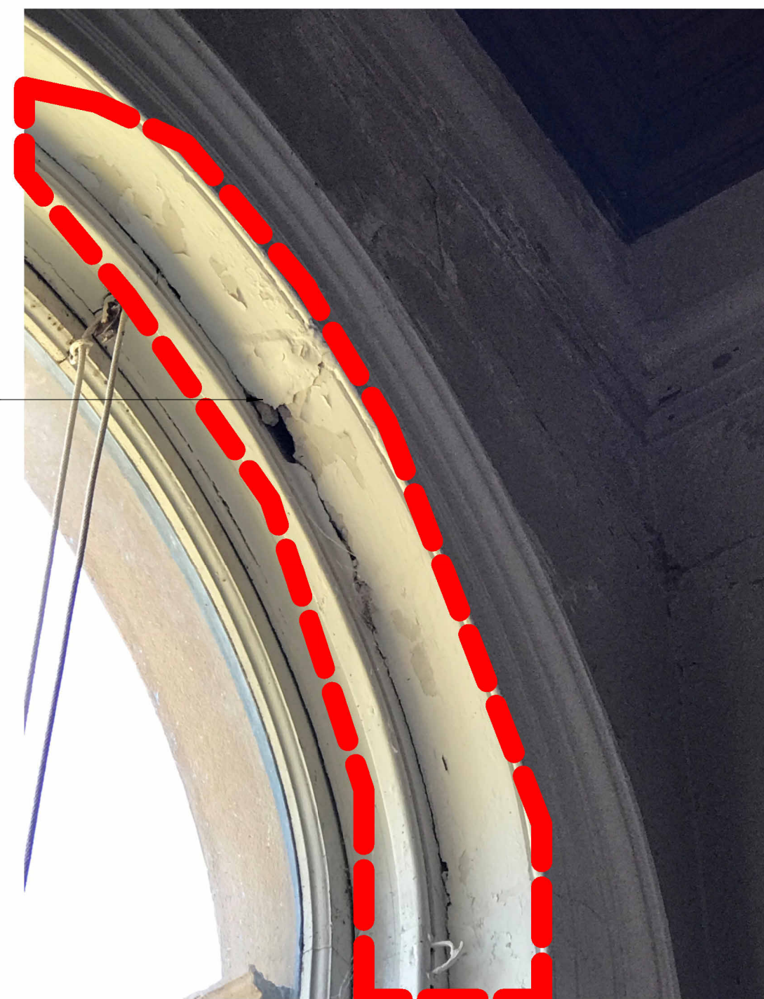
Repair and restore existing decorative moulding. Moulding to match existing profile.
