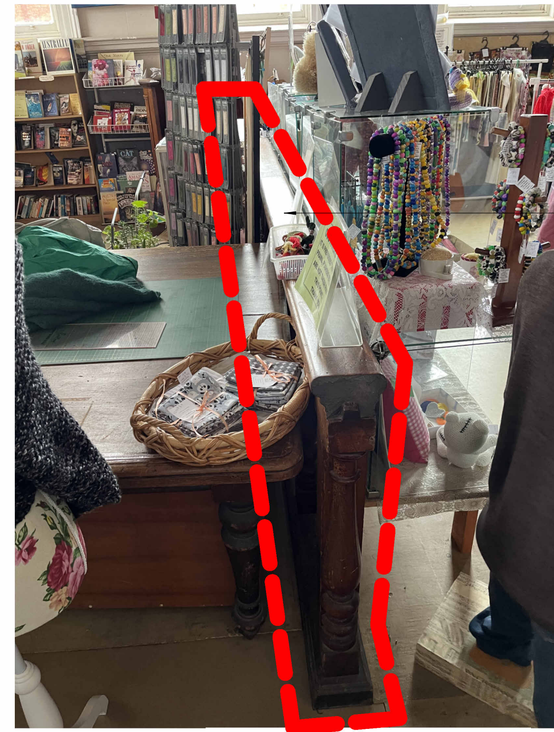
Restore existing timber decorative handrail, light sand and re-oil to match existing colour tone.
