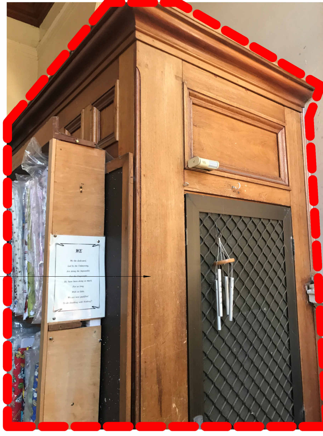
Restore existing Judge desk and clerks desk, removed existing vinyl flooring and make good as require. light sand and re-oil to match existing colour tone.
