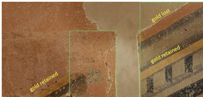
Figure 12 Composite view of the 1990s paint removal efforts. It can be seen that where gold is retained well in some cases, it has been completely removed in others.
