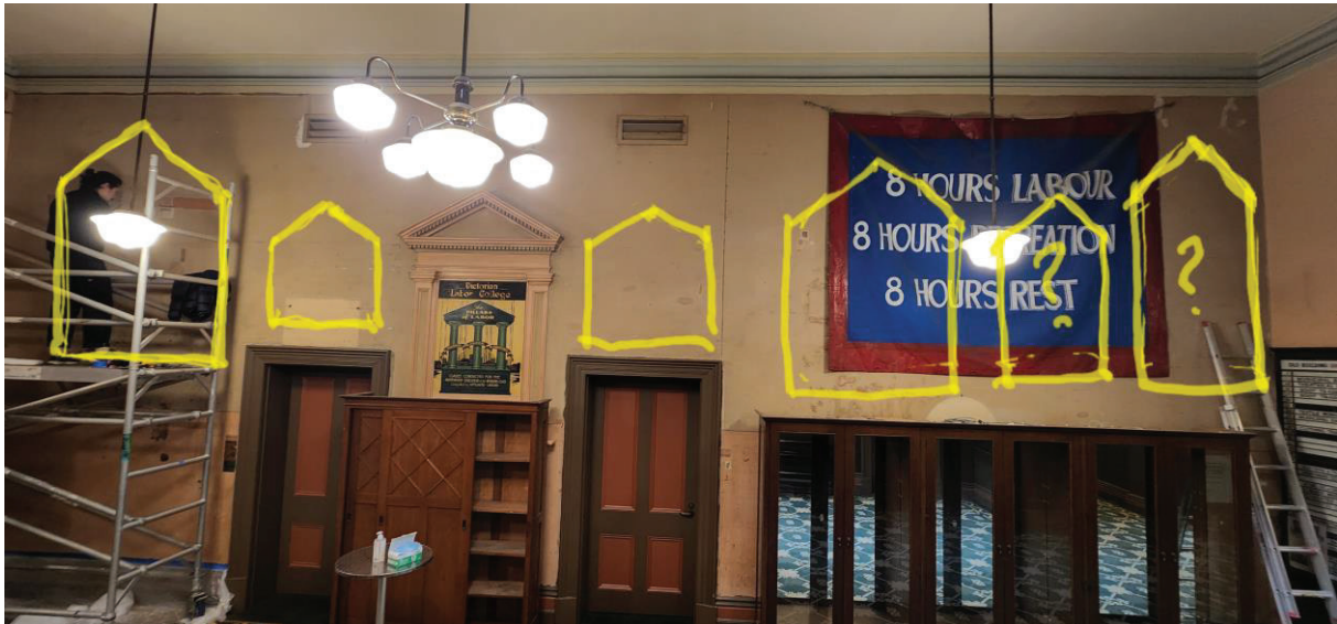
Figure 7 Raking light has confirmed plaques in the layout suggested in this markup.
