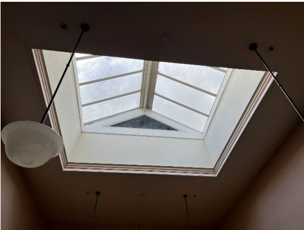
Figure 12 Typical skylight viewed from viewed from F34
