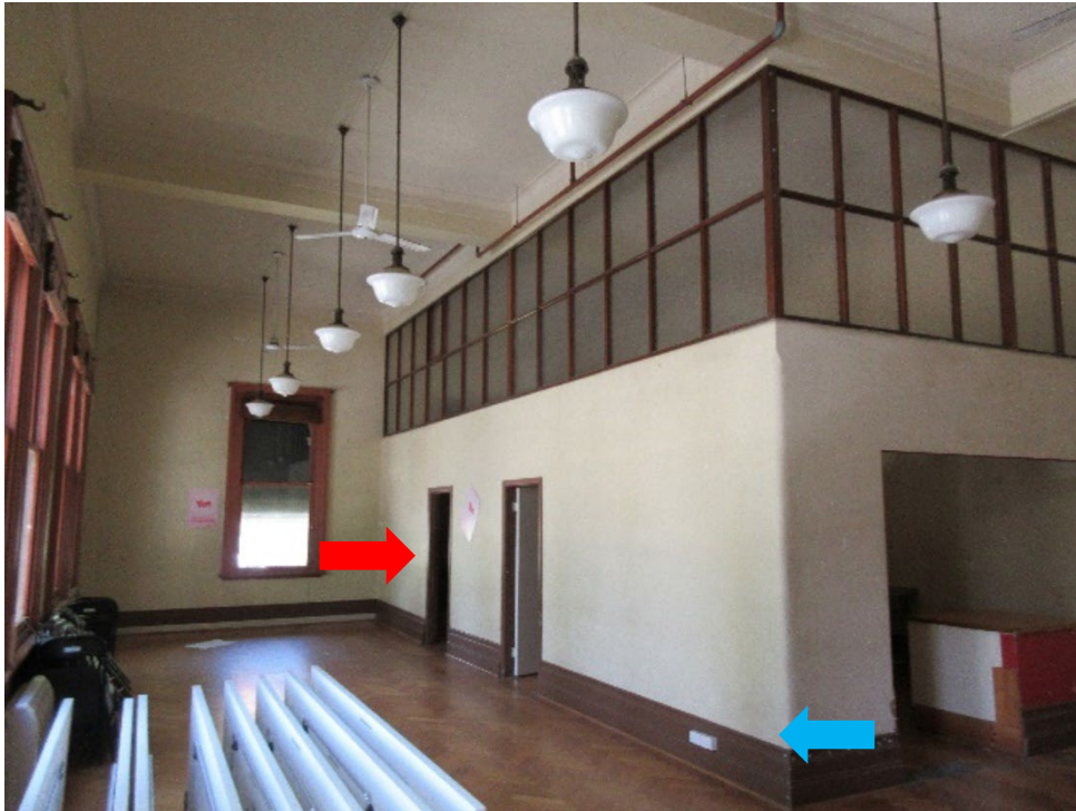
Figure 13 Layout of G39 proposed for reconfiguration to create offices; red arrow indicates door opening to be infilled and skirting; blue arrow showing location of proposed lightweight wall to extend to perimeter wall
