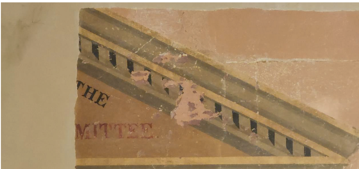
Figure 14 Paint removal areas on the west wall.
