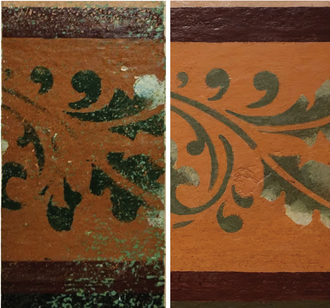
Figure 10 Comparison between the original stencil on the west wall (right) and the extant stencil on the east wall. It is noted that the highlighting of foliage on the east wall is absent from the exposed original on the west wall.
