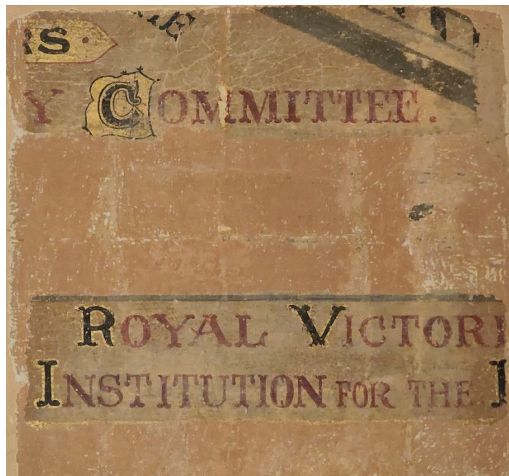
Figure 5 Raking light on the south wall has revealed a plaque either side of the opening. A rough repair to the previously ruled ashlar in the plaster can be seen as can the faint linear outline of the pediment to the western plaque.
