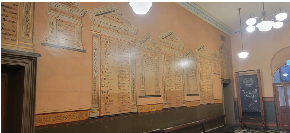
Figure 1 General view of the East wall.
