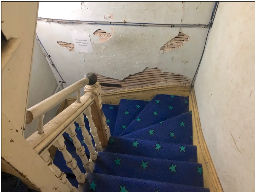
Figure 22 View from the second flight of stairs, 2022.
