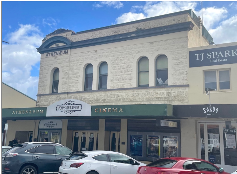
Figure 8 The Athenaeum façade prior to the restoration works, 2022.
