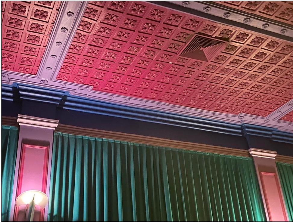
Figure 18 The decorative plaster ceiling in the main auditorium with c1990s colour scheme, 2022.
