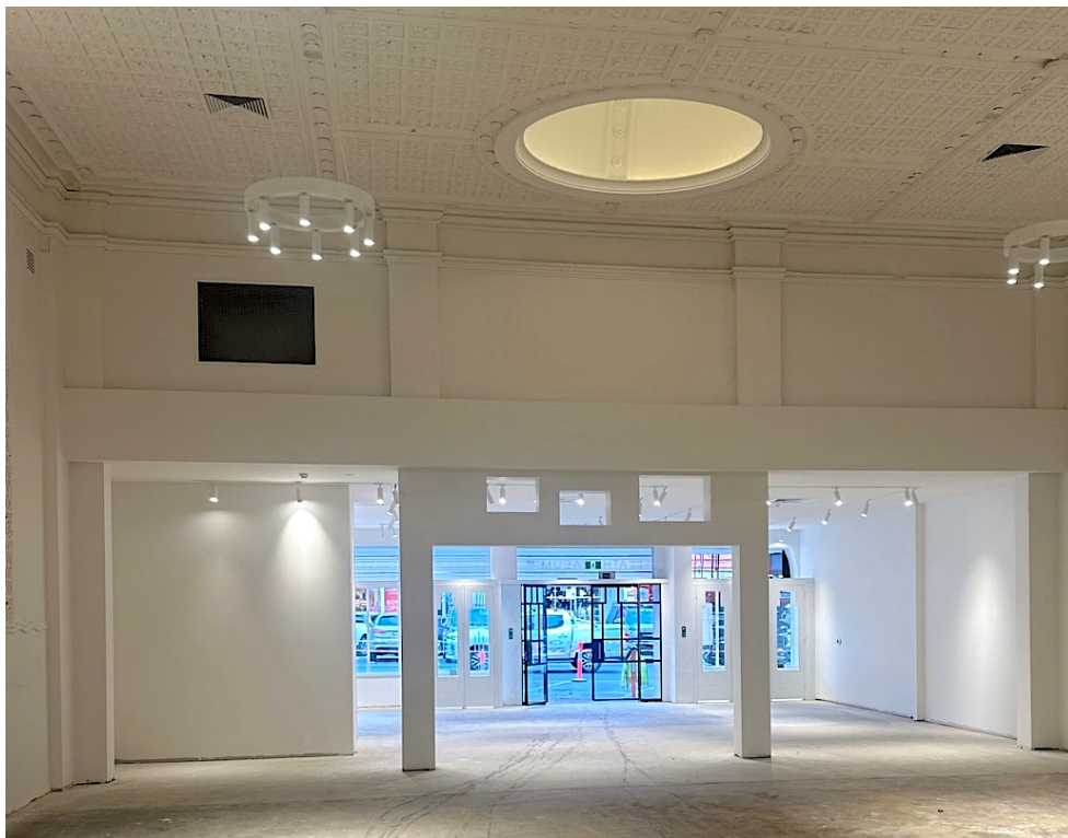
Figure 17 The south wall of the restored auditorium with retained bio-box apertures. The stair enclosure is visible to the far left.
