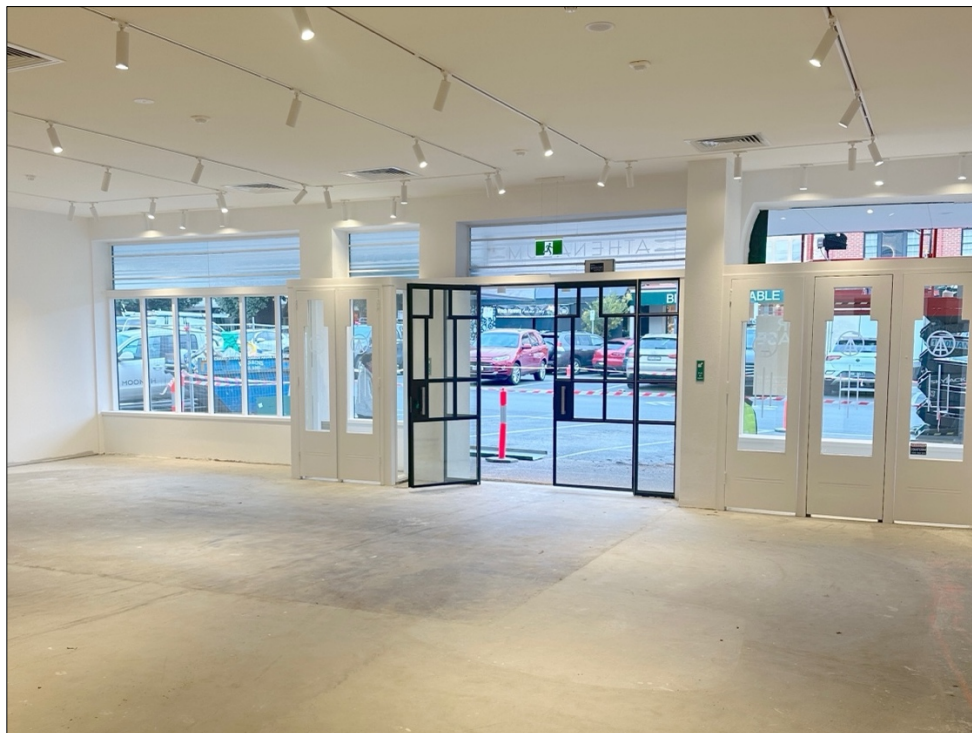
Figure 11 Recent photograph of the foyer showing the new entrance with Art Deco style doors reinstated to the interior of the shopfront as interpretative features.
