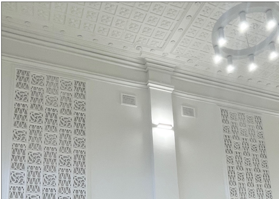
Figure 19 Detail of the restored ceiling and plasterwork.
