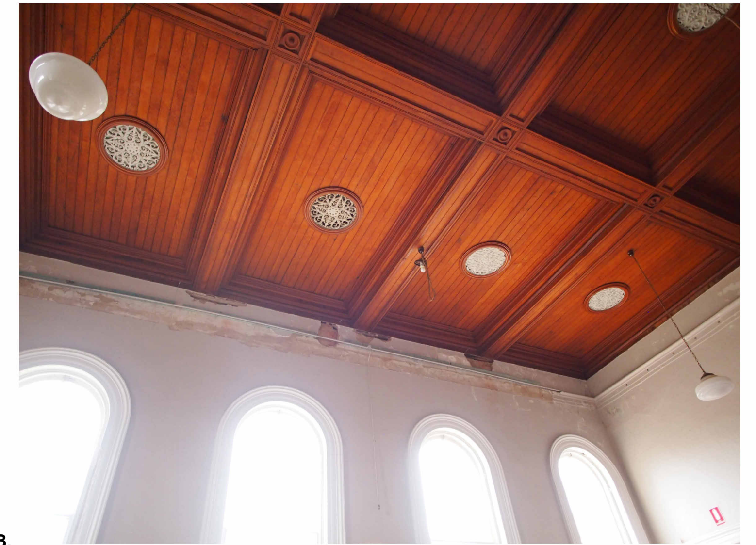
B. Repair hard plaster and decorative plaster rail detail above windows to match existing.
