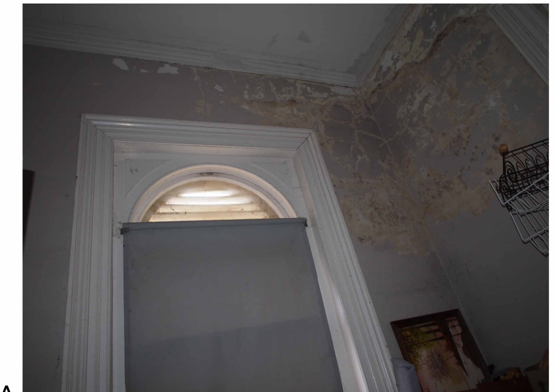
A. Repair and make good all internal wall linings to match existing and provide new paint finish throughout building. A. Colours typically to match existing
