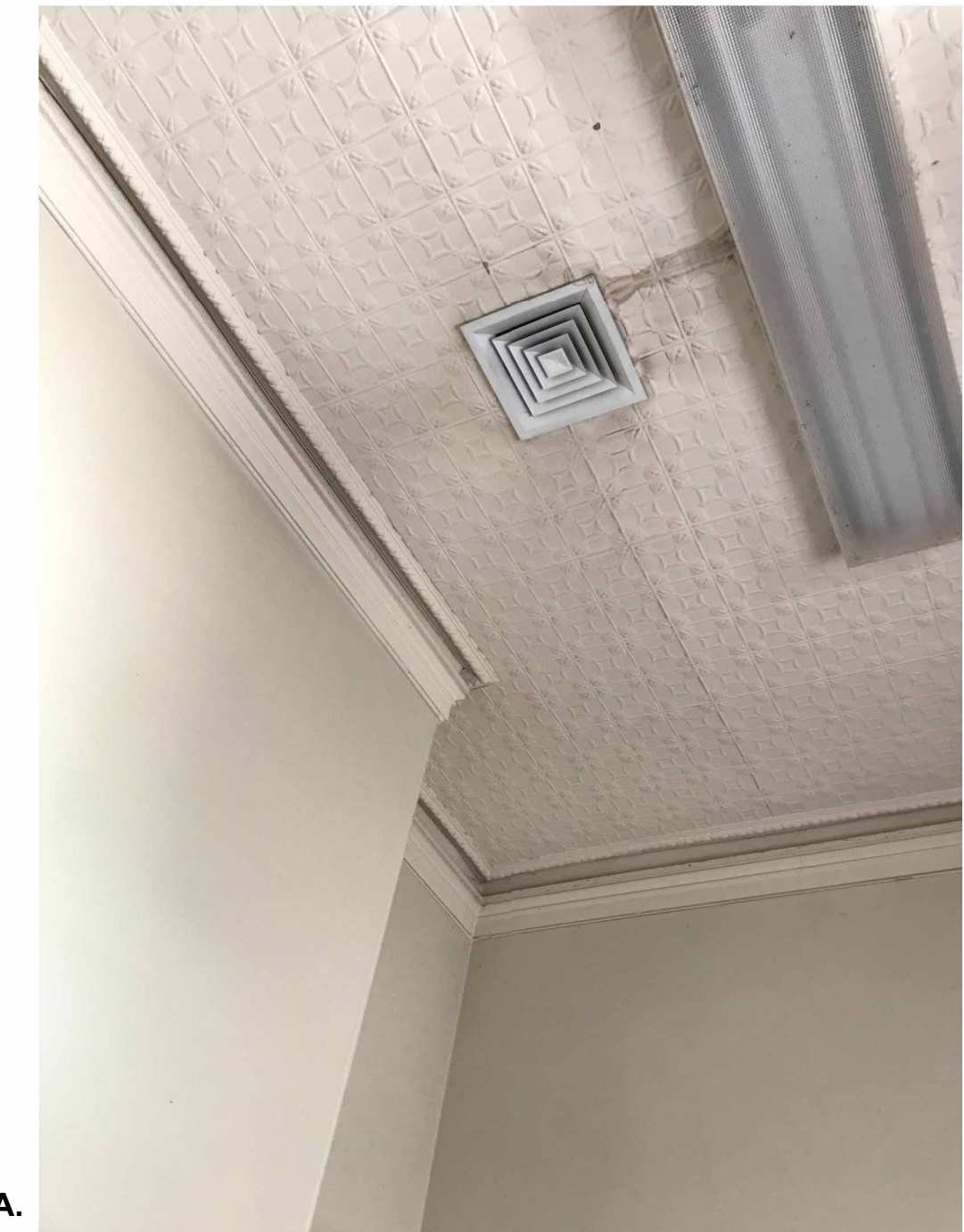
A. Clean and paint existing pressed metal ceilings throughout building. Colour to match existing
