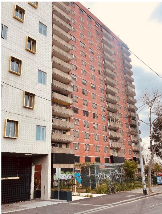
August 2024, No. 141 Nicholson Street, east elevation viewed from Nicholson Street Source: Heritage Victoria.
