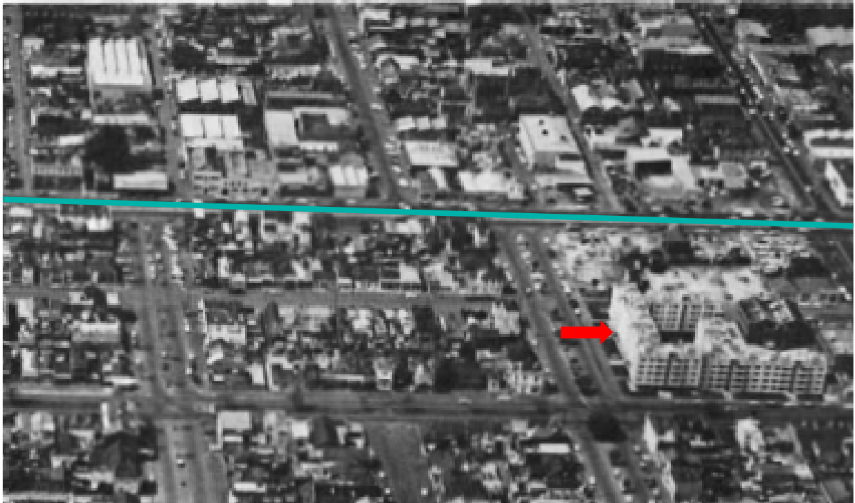
1964-65. View of Carlton prior to the construction of the Nicholson and Elgin Street Towers, looking east towards Fitzroy. The walk-up blocks at the Palmerston Estate are indicated with a red arrow. Nicholson Street is shown in teal. Source: Housing Commission of Victoria, Annual Report, 1964-65, p. 10. Reproduced in Exclusion Application.
