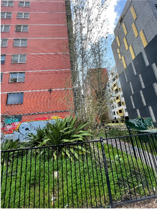
August 2024, View from Elgin Street. Shows 20 Elgin Street (front LHS of photo), 141 Nicholson Street (middle of photo at rear) Source: Heritage Victoria.
