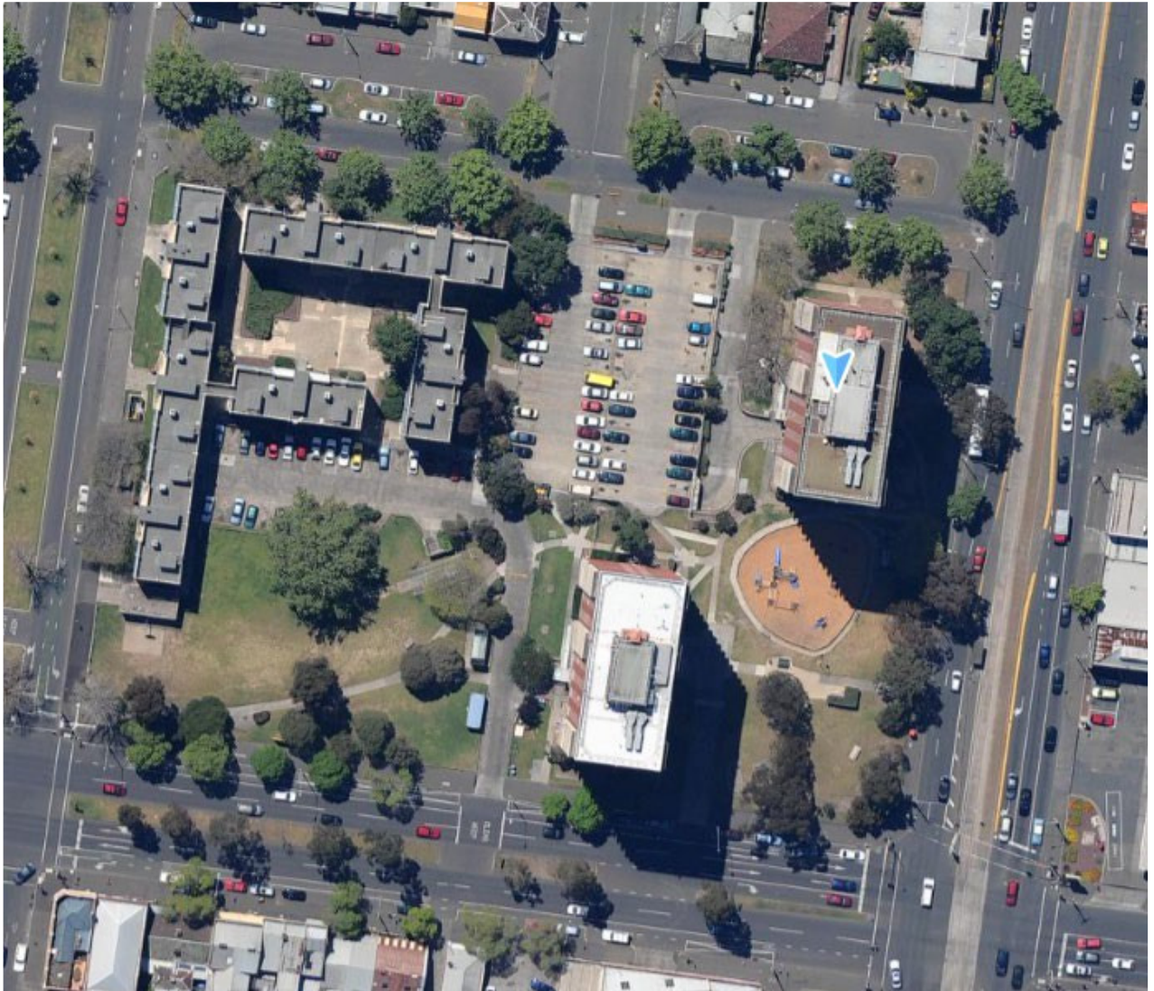
Satellite imagery from 2009. The Nicholson Street Tower is denoted with a blue arrow. Reproduced in Exclusion Application.
