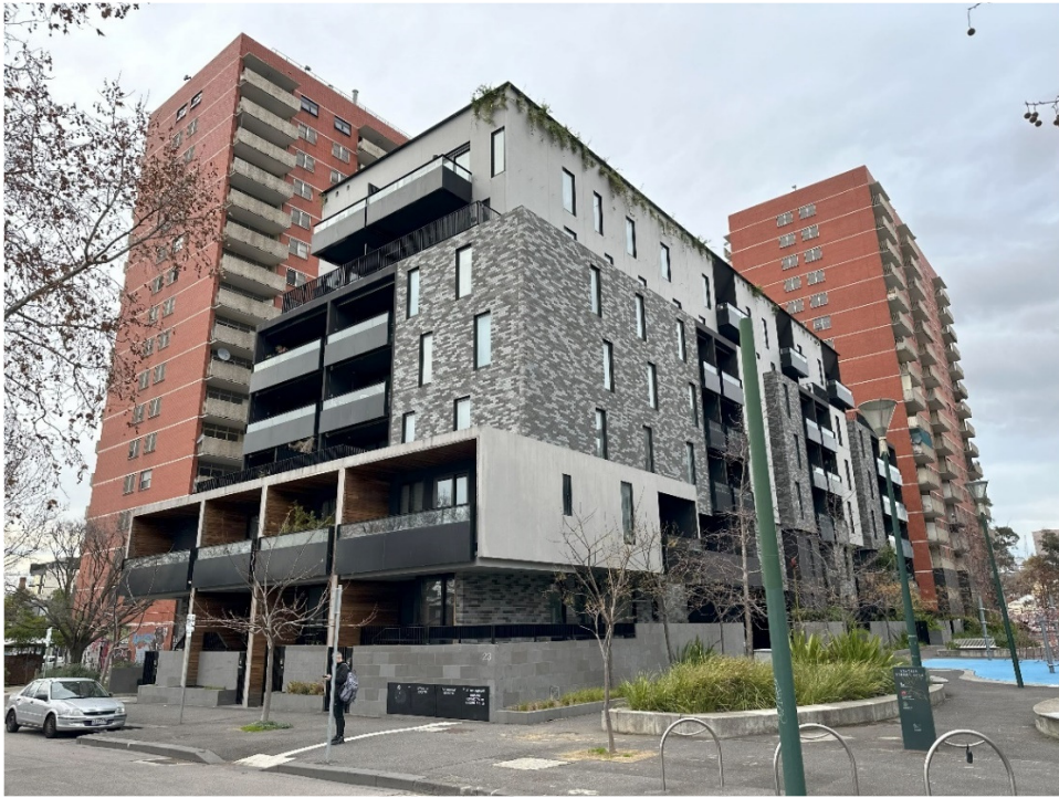
August 2024, View towards the southeast from the corner of Canning and Palmerston Streets Source: Lovell Chen.
