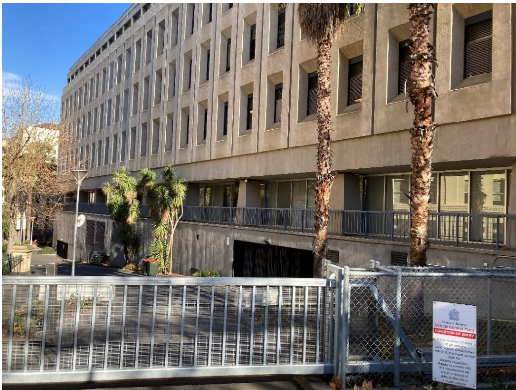
Figure 10 East elevation and basement level entry, view from St Andrews Place
