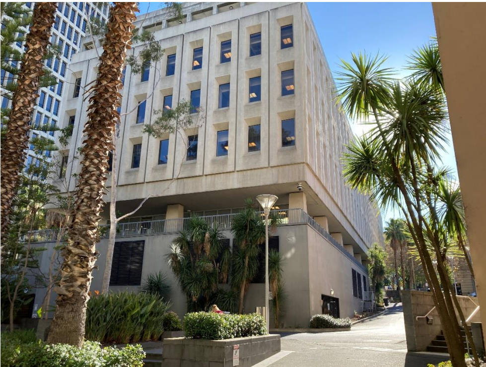
Figure 8 View from within the Treasury Reserve to the south and east elevations of the building
