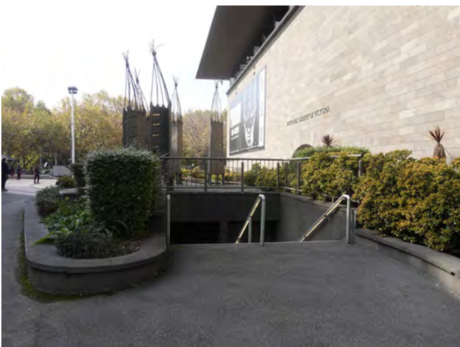
Fig 18: View of current fire-egress stair and gardens to North Elevation of the NGV International Main Gallery Building, looking east (Purcell, 2024)
