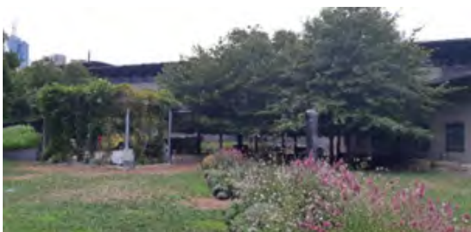
Fig 41: View looking north-east, toward the West Elevation of the NGV International Main Gallery Building with the Arts School to the left.
