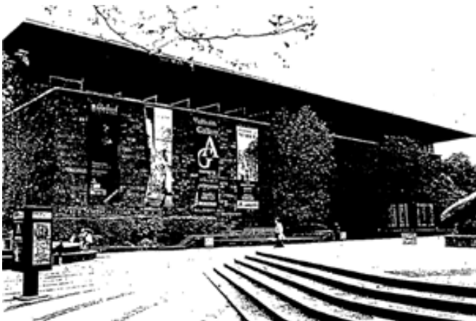
Fig 24: North elevation 1997, compromised by the loss of the moat (Figure 65, NGV CMP Meredith Gould Architects, 1998).
