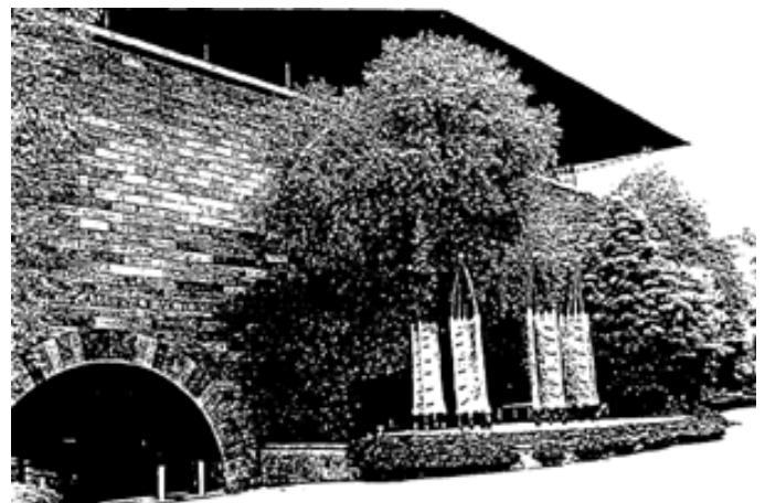
Fig 25: North West view, 1997. Note the raised planter in lieu of the moat here and the sloping ground towards the "mousehole" to accommodate the raised level for the State Theatre (Figure 90, NGV CMP Meredith Gould Architects, 1998).
