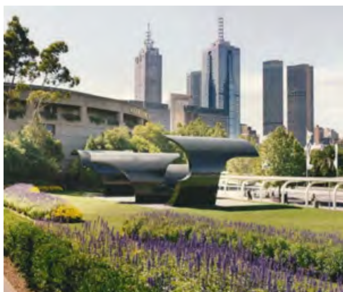
Fig 33: View from south-west c.1981 with original landscape treatments, including eucalyptus trees to south of the Concert Hall. (Source: National Trust – Trust Advocate) 15
