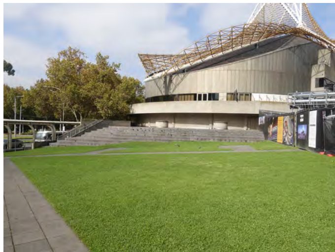
Fig 11: View of North Elevation Theatres Building, across Arts Centre Lawn (Purcell, 2024).
