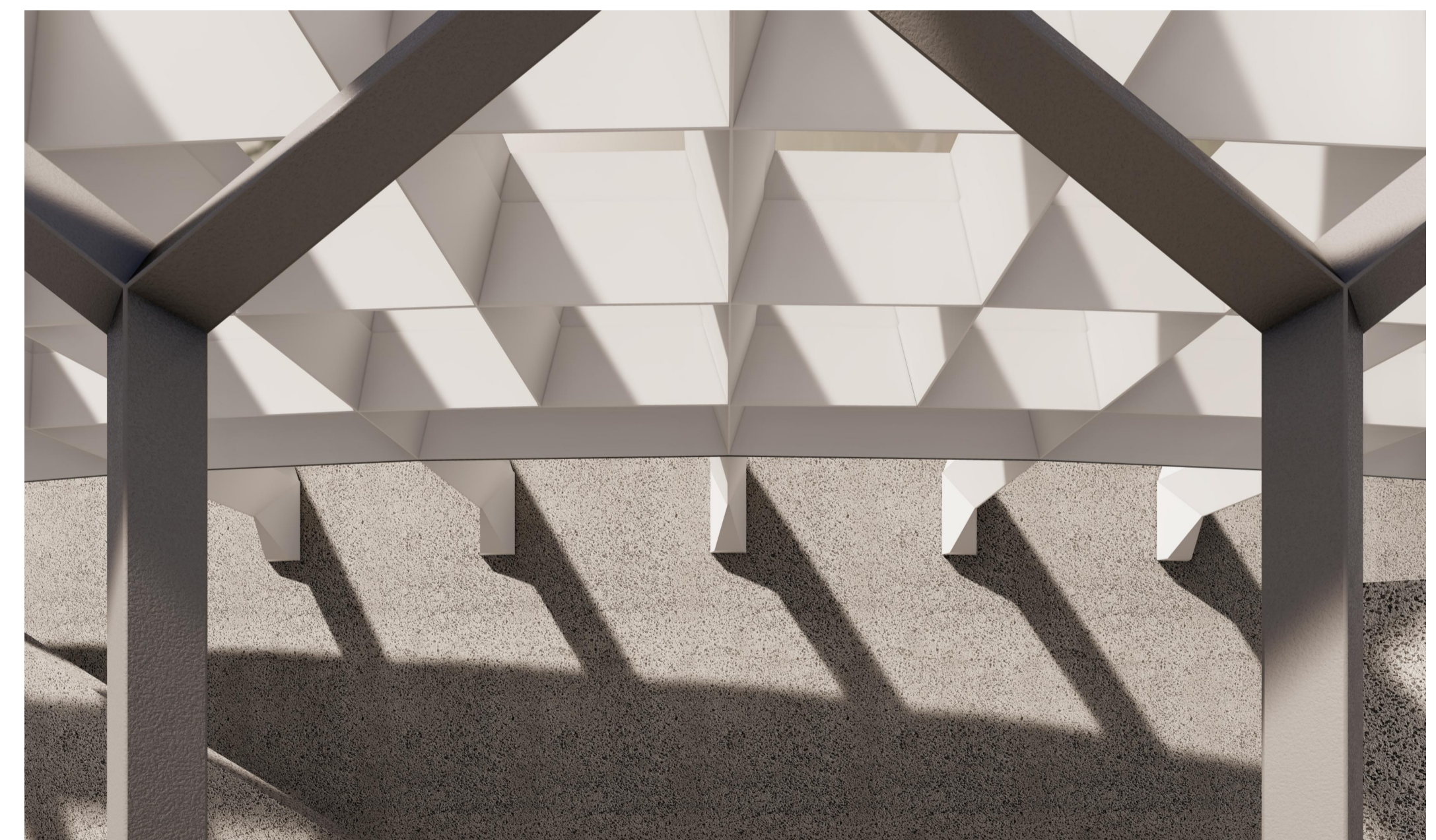
WESTERN CANOPY | PROFILED BEAM DOWNTURNS
