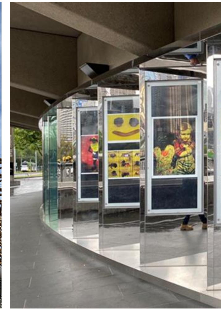
The more recent addition of frameless glazing at Hamer Hall by ARM.
