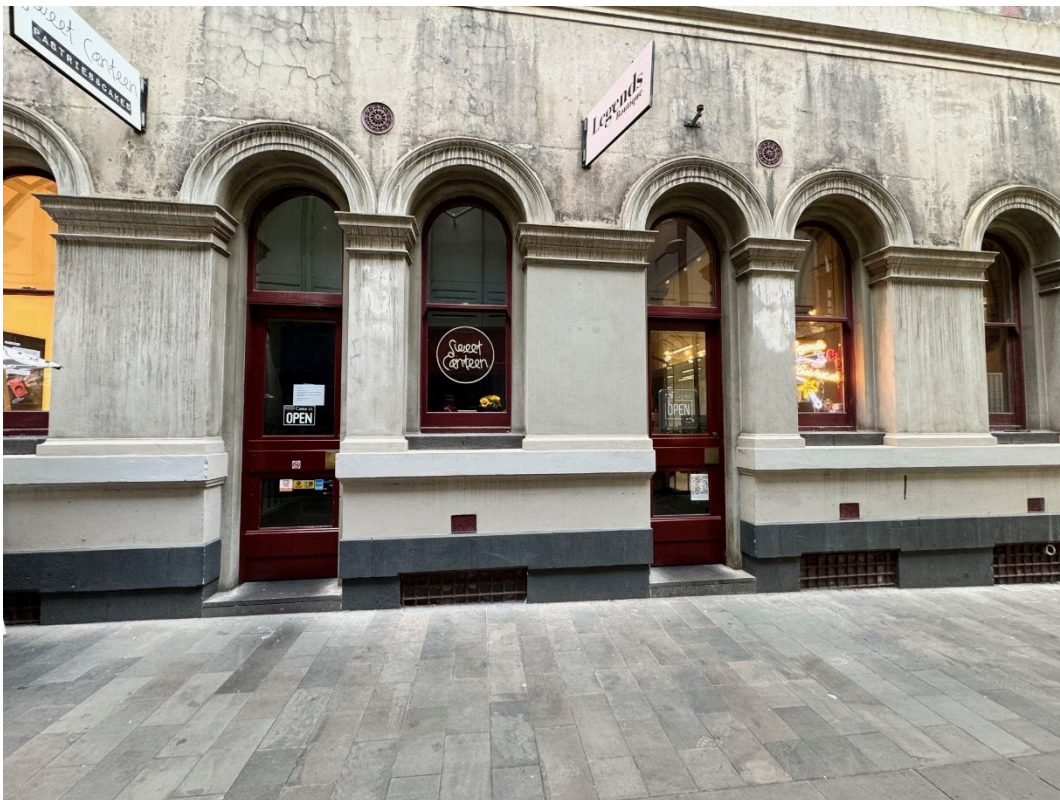
Conversions of original windows into doorways (Shops 2 & 3)
