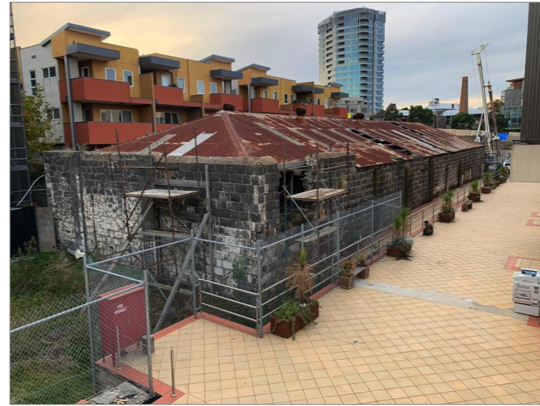
PHOTO 3 - REAR SOUTH ELEVATION WITH COURTYARD
