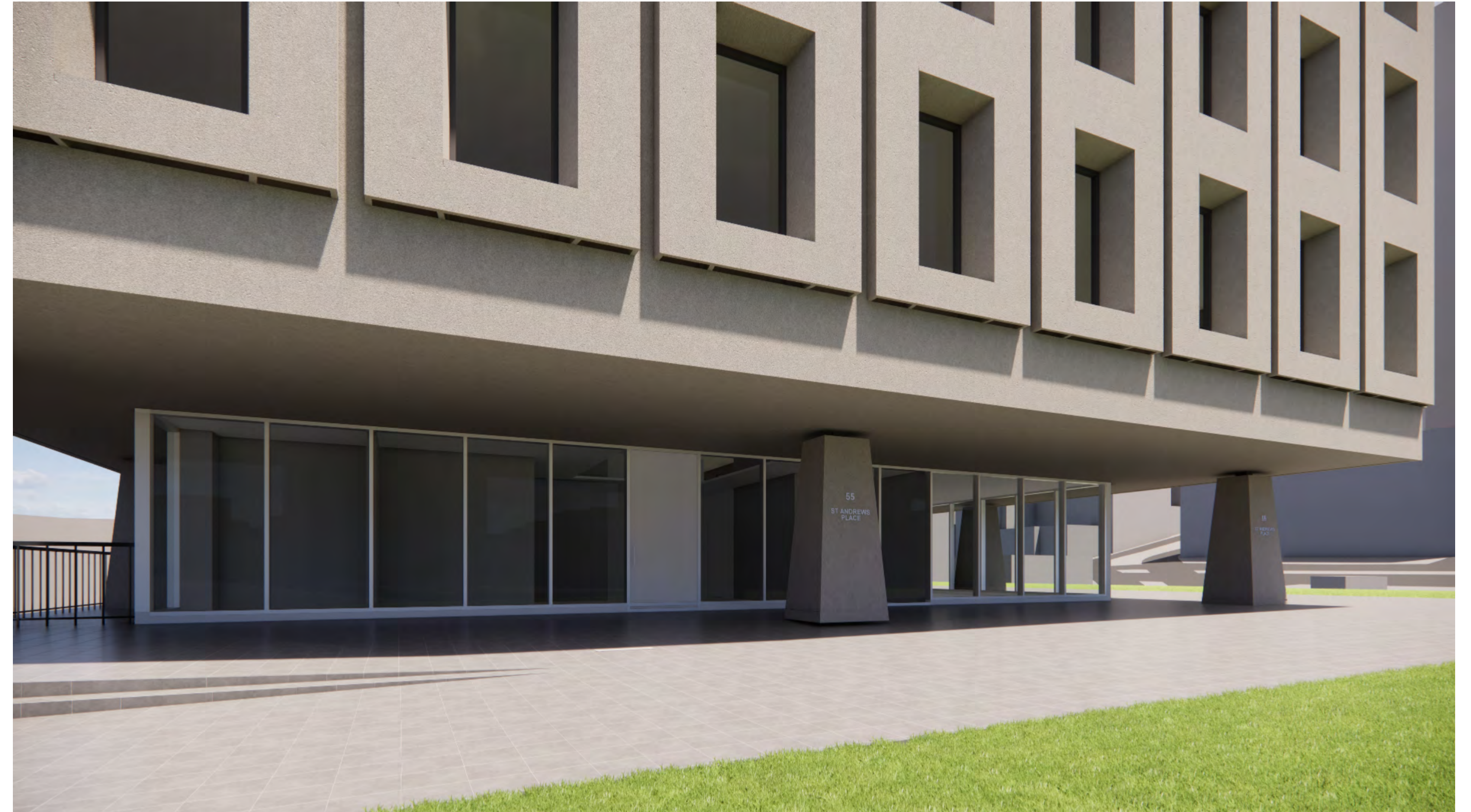
VIEW 2 - SOUTHERN VIEW FROM ST ANDREWS PL (EXISTING)
