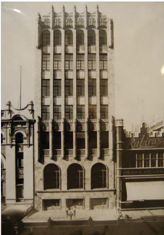
Subject building - eastern section built in 1929-30 (Source: SLV, Manuscripts Collection)
