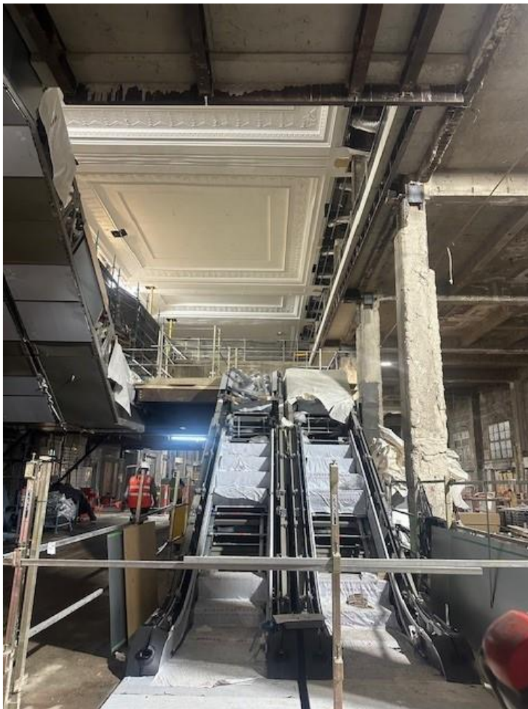
Ground floor level – new void/mezzanine and escalators (photo courtesy of MECCA)
