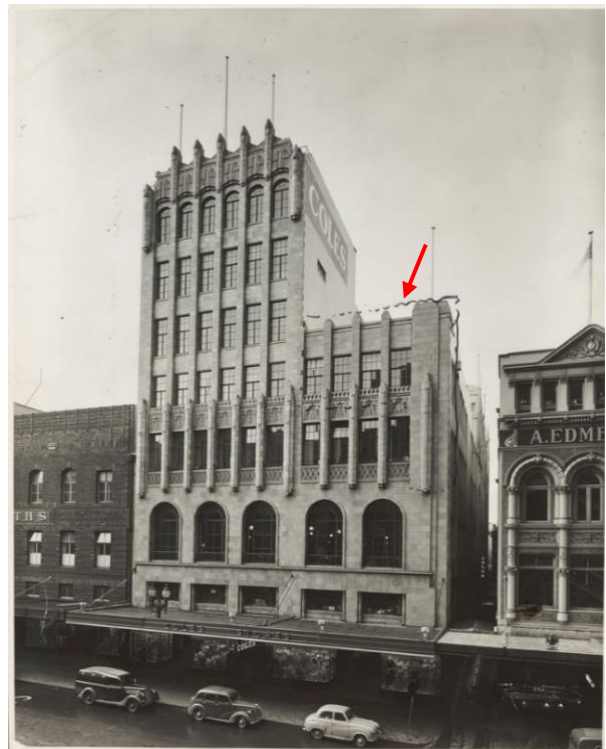
Western addition built in 1939, with new canopy (Source: SLV, Records of Coles Myer Ltd.)
