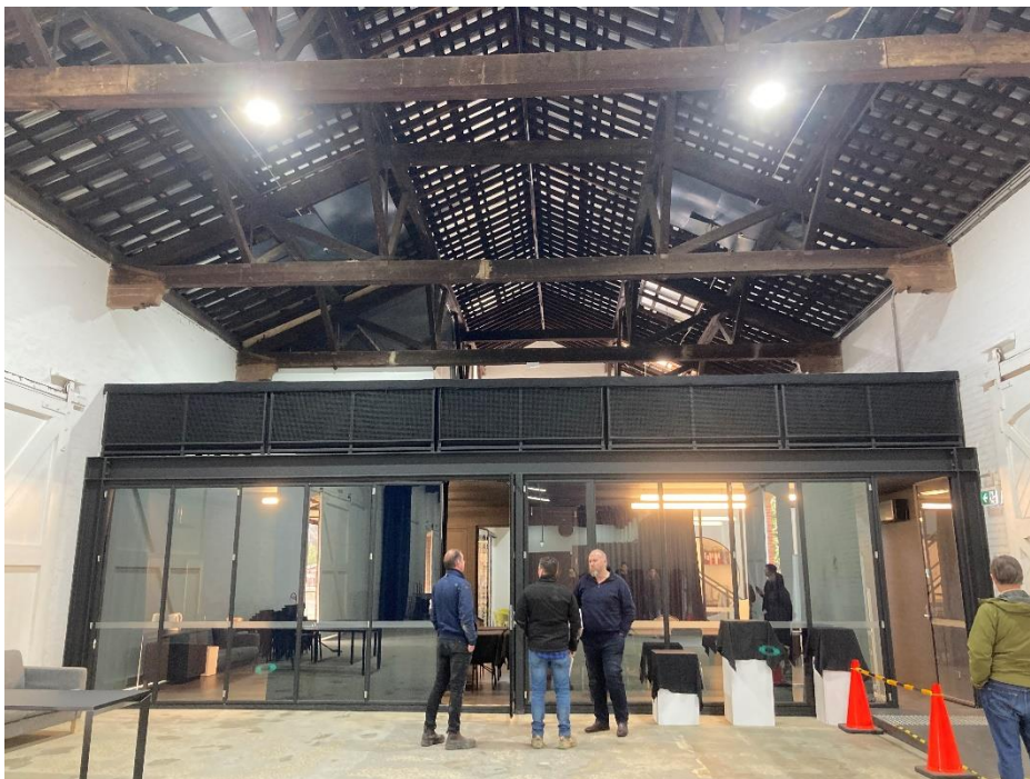
Ground floor level – new void/mezzanine and escalators (photo courtesy of MECCA)
