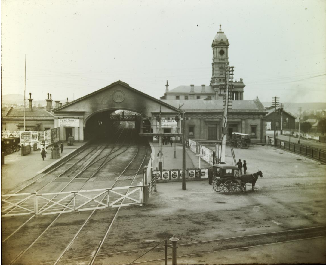
Figure 6 Photograph showing the sector gates (gates 3 & 4) at Lydiard Street North, looking south-east towards the station, c. 1890s
