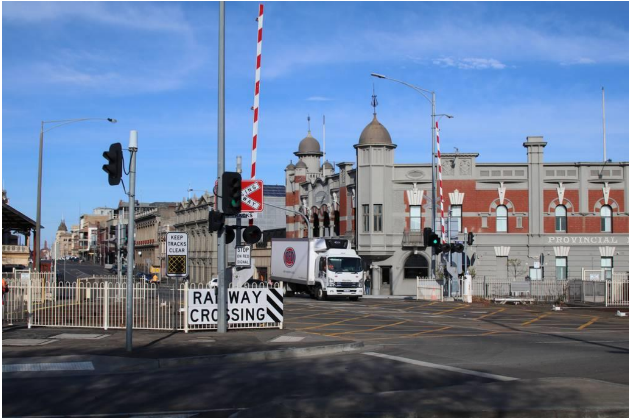
Figure 5 Road Crossing Overview
