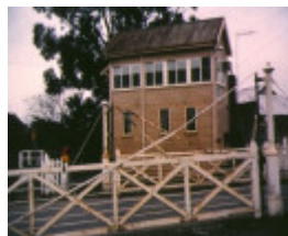
ballarat railway complex signal box & gates
