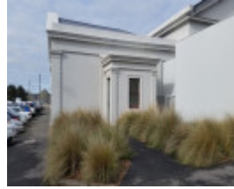
Reconstructed entry porch, north side station building refer P20705
