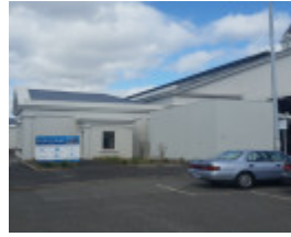
Reconstructed entry porch to the north side station building refer P20705
