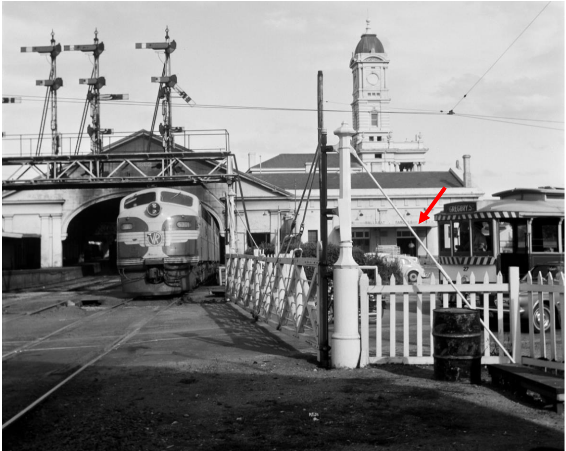
Figure 7 1967 view of the Lydiard Street crossing, note the addition of a second tie rod attached to the gate and supporting rod (red arrow) Source: State Library of Victoria, H83.156/195
