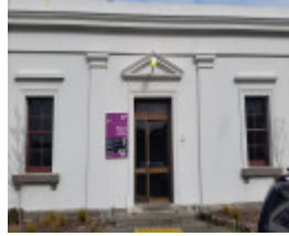
Modern and highly intrusive entry door to the north side station building
