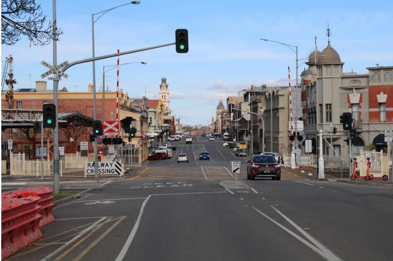
Figure 6 Road controls (northern approach)
