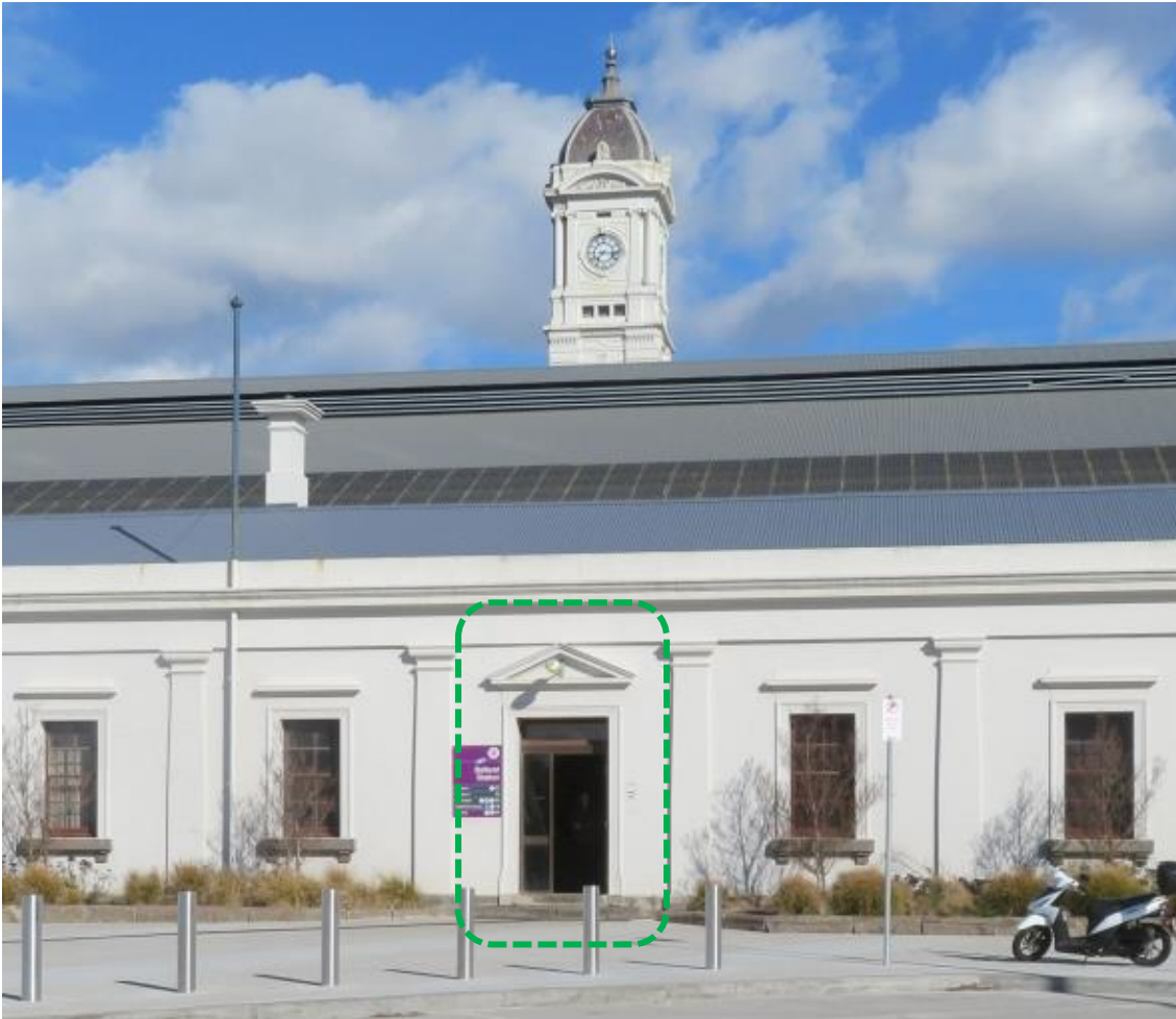
Figure 4 Non-compliant entry to the North Station Building, indicated
