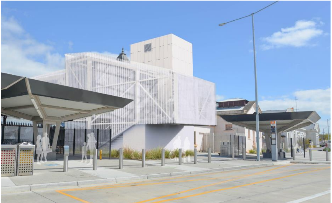
Figure 20 Visualisation of the stair and lift core on the north side of railway station Source: LXR and WPA documentation WSP-712-D-WPA-M3D-67-BAT-ARC-0000H
