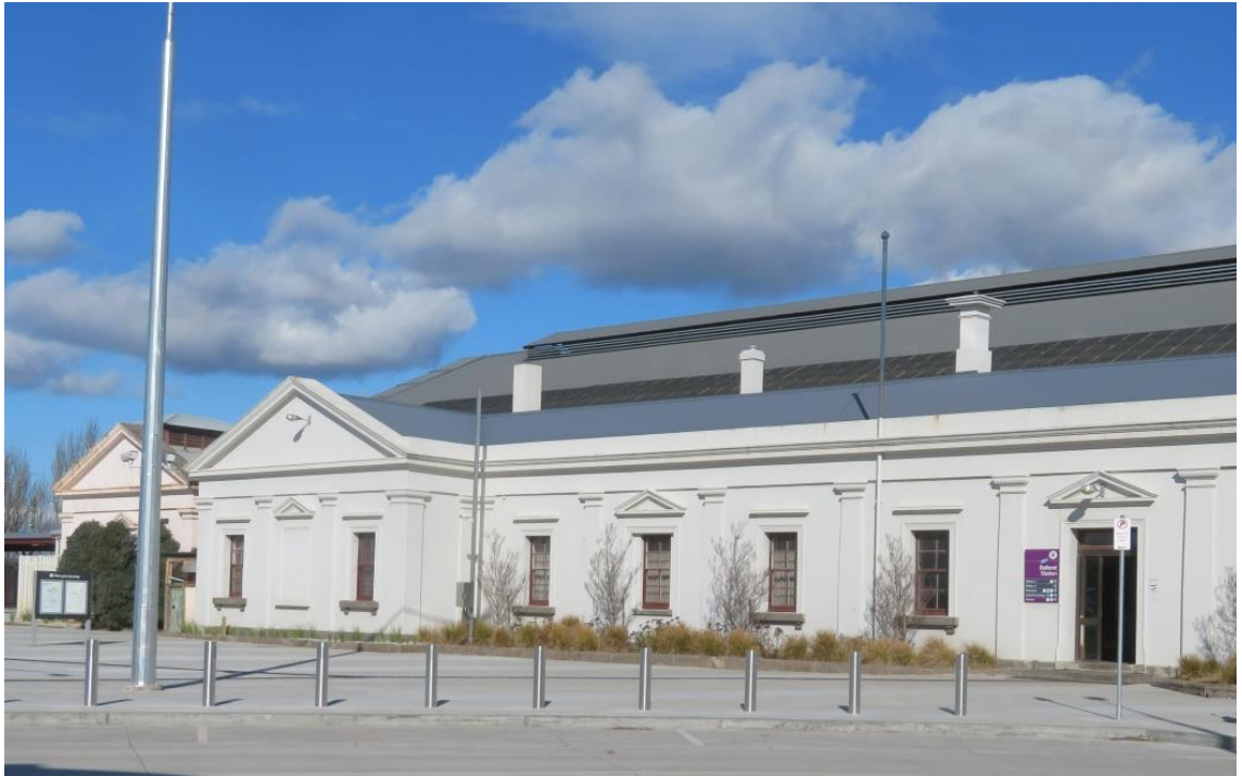
Figure 14 View of the west half of the north elevation of the North Station Building
