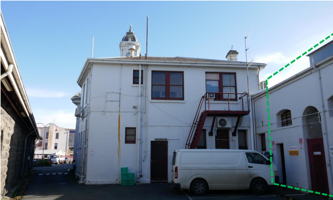
Figure 13 View looking west: the east wing of the South Station Building is at right: the indicative extent of the elevation that will be demolished is indicated
