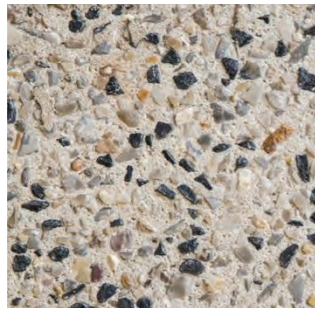
POV-02 Exposed Aggregate seeded with contrasting colour
