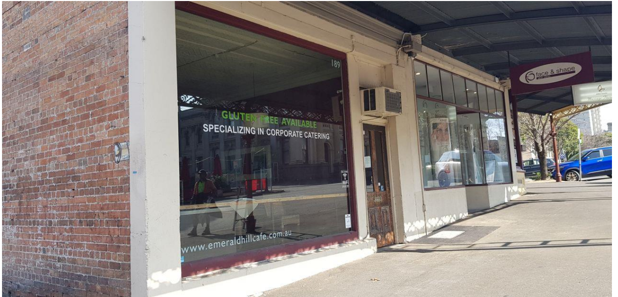
Figure 14 Ground floor shopfront of 189 Bank Street
