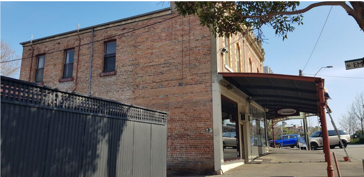
Figure 13 East elevation of 189 Bank Street
