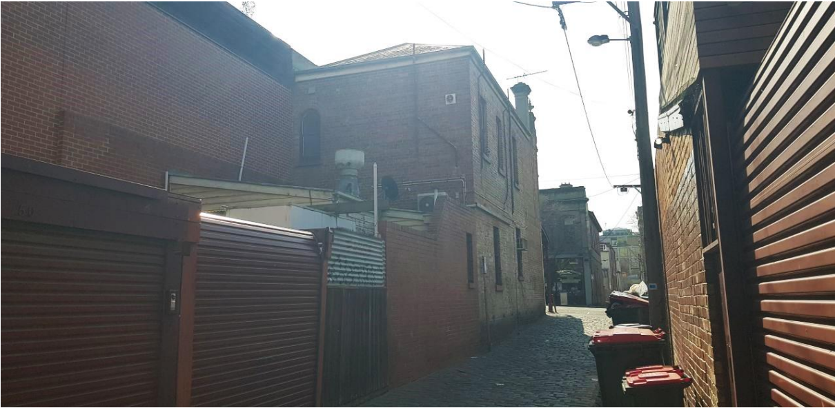
Figure 16 Rear wall of 189 Bank Street with round headed window visible above single-storey weatherboard wing and roller doors to Emerald Hill Place
