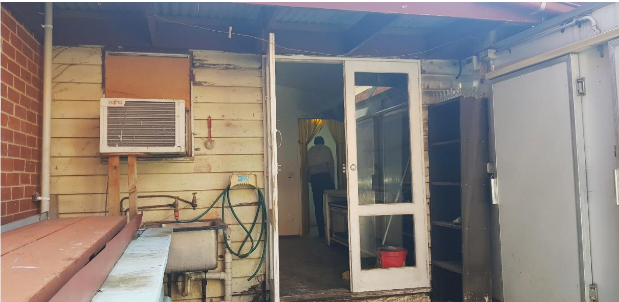
Figure 17 Rear weatherboard wing
