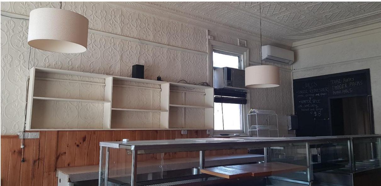
Figure 19 Pressed metal to walls, cornice and ceiling
