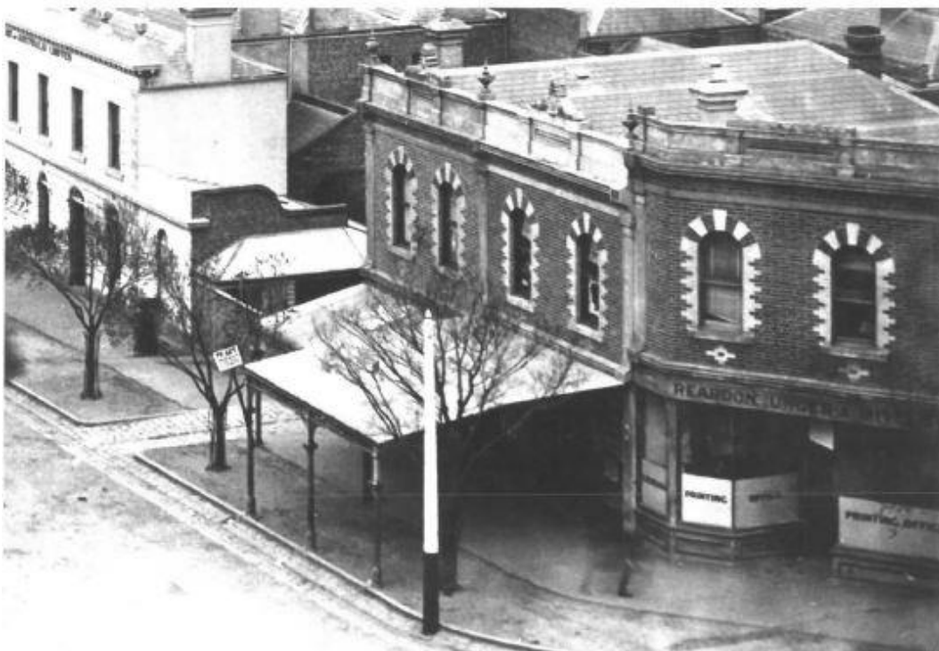
Figure 6 1889-90, David Wood, Oblique aerial of 189-193 Bank Street Source: Emerald Hill Estate: Conservation Study and Policy , 1983
