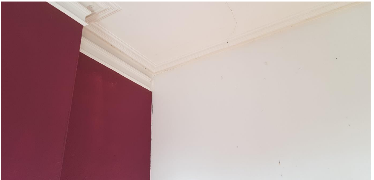
Figure 22 Original cornice of master bedroom terminates at introduced wall
