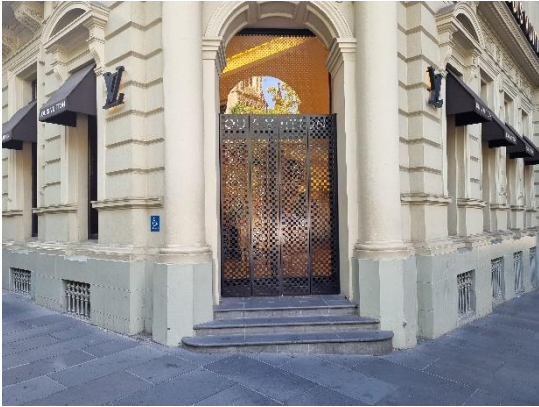
Figure 15 Security gate to 139 Collins Street (HO577, HO504)
