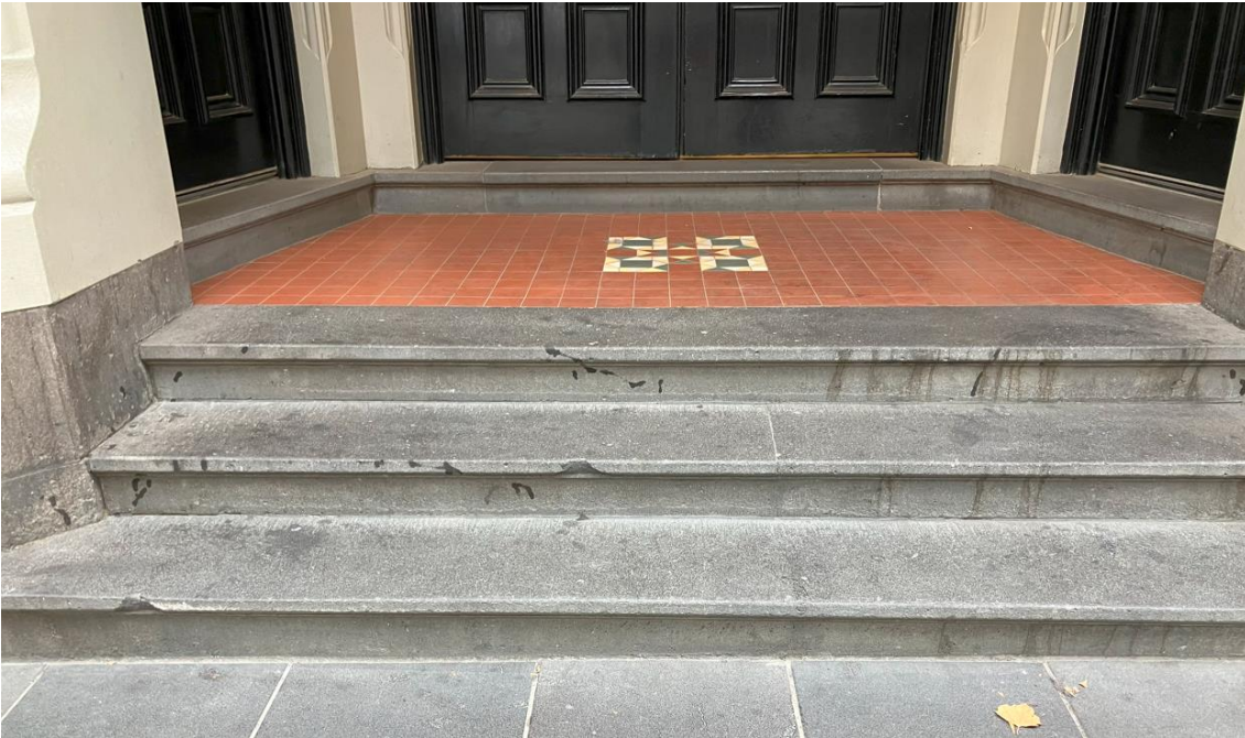
Figure 11 The existing front entrance steps
