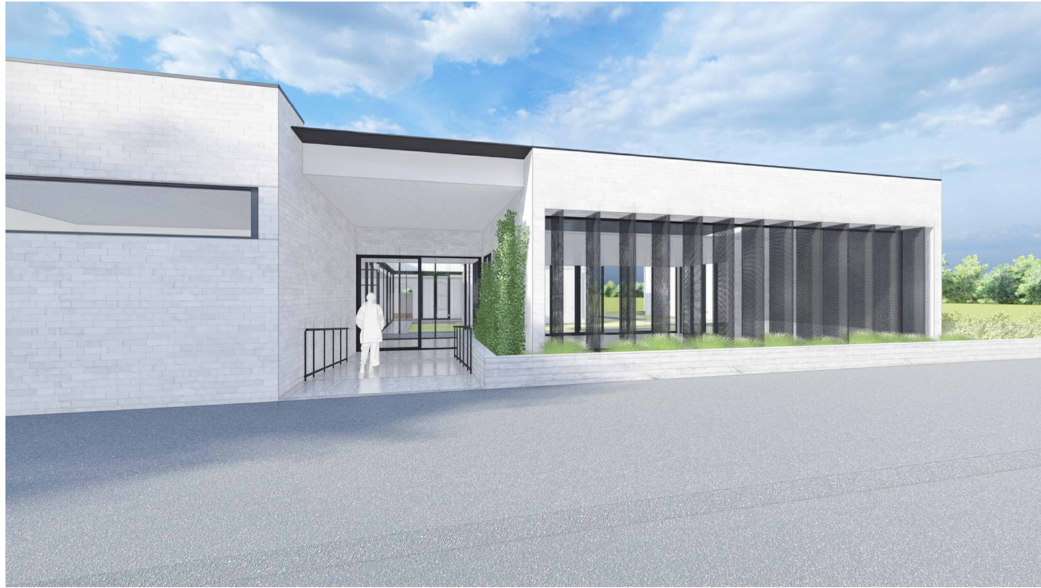
Rotatable sun shading element devices Open - Winter setting
