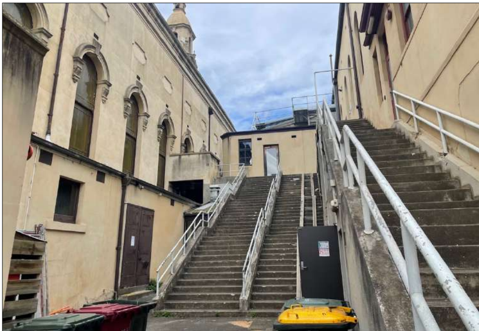
Figure 24 The rear service yard showing concrete stairs erected c1938.
