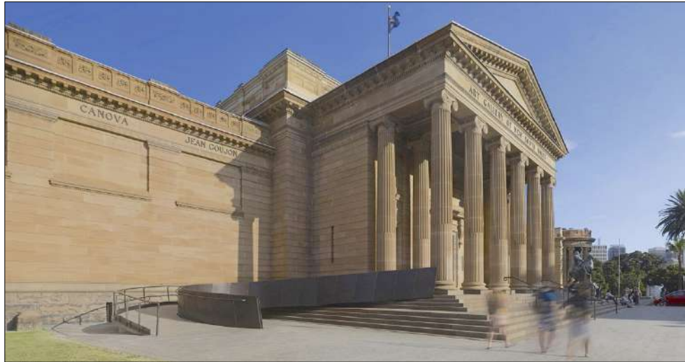
Figure 35 DDA access ramp to the front of the Art Gallery of NSW.
