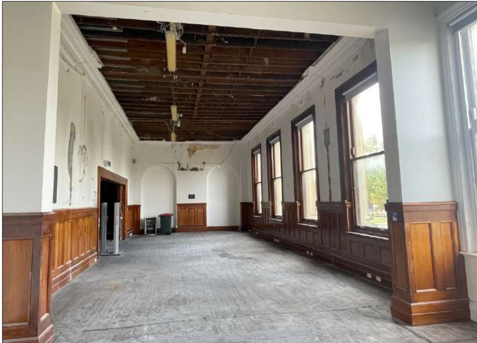
Figure 29 Former Council offices/lounge on the ground floor, looking east.
