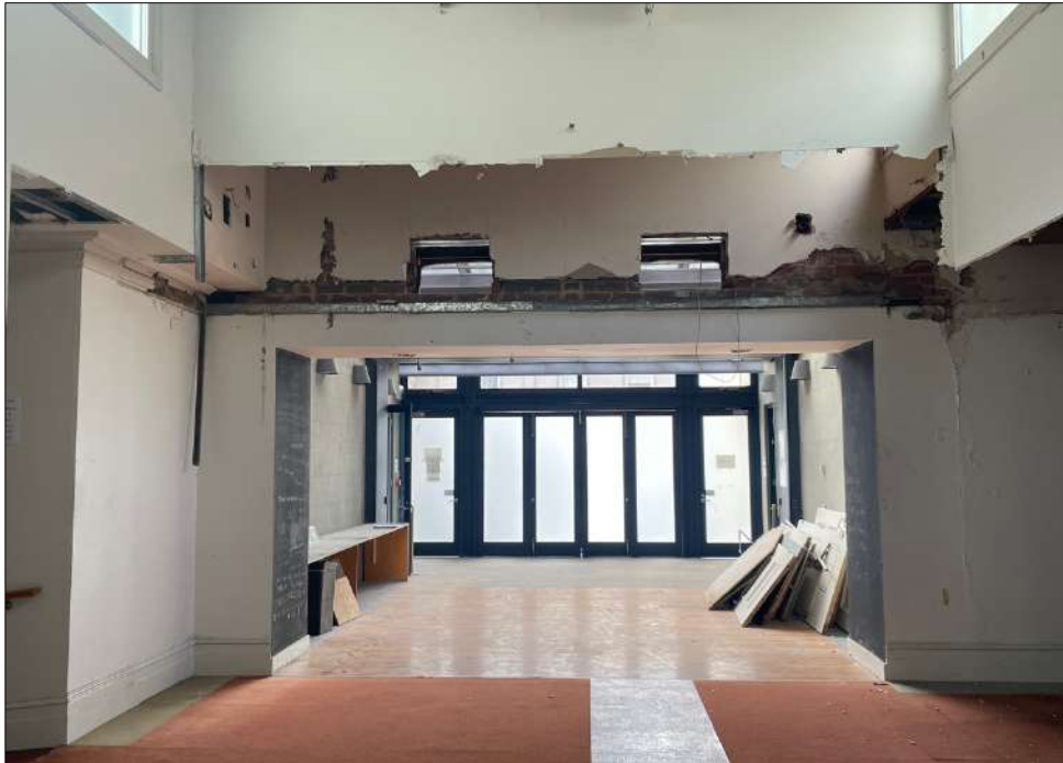
Figure 31 Altered foyer space on the east side of the main hall.
