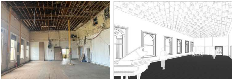
Figure 51 (left) Former supper room looking west.
