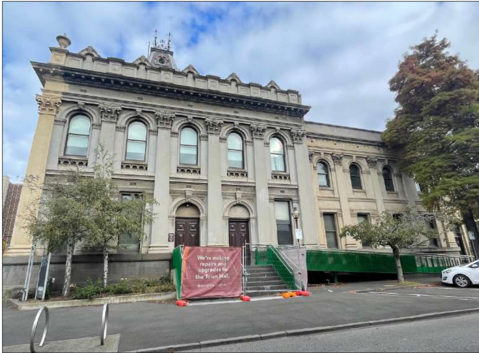
Figure 19 The southern half of the east elevation.
