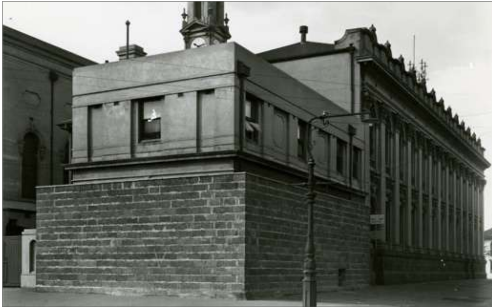
Figure 14 A c1945 photograph showing the first floor assistant librarian's flat. Note the ground floor enclosed by a masonry wall – presumably because it housed an x-ray clinic at this time. Source: Port Phillip City Collection.
