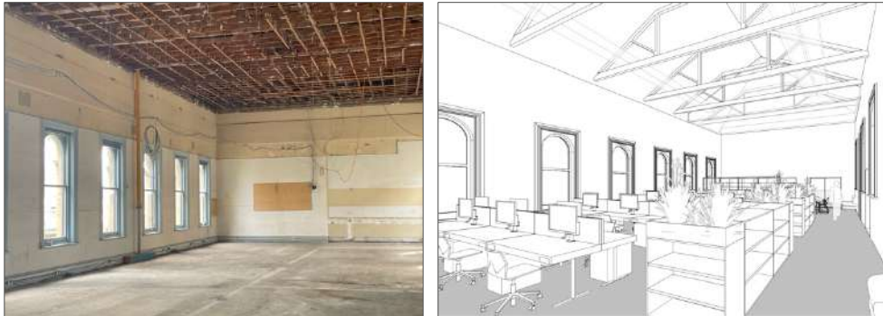
Figure 53 (left) Former lodge room looking north.
