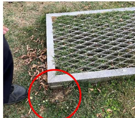
Figure 3: Example of the fixing mechanism for the walkways. The relocatable Pontoon will use a double walkway, pinned as shown and in accordance with the specifications provided in section 8.
