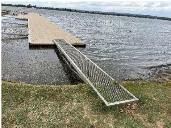
Figure 3: Example of the fixing mechanism for the walkways. The relocatable Pontoon will use a double walkway, pinned as shown and in accordance with the specifications provided in section 8.
