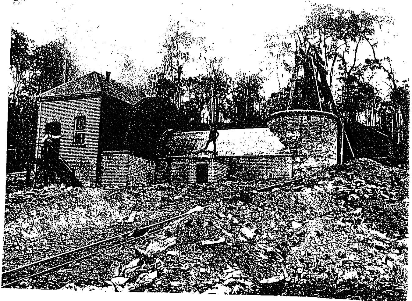
Ventilation fan house at Seaham Colliery, Hunter Valley. Engine house to left, then circular fan housing to left of the person on the roof, and air shaft and headframe to right. Inclined tramway in foreground. (NSW Mines Department Annual Report 1900)
