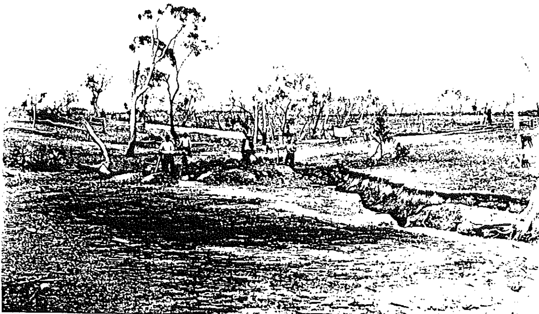
Shallow sinking (pot hole tailings), the most basic form of alluvial mining, near Murrumburrah, NSW
