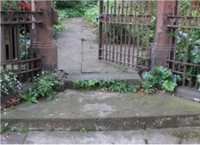
Figure 14 Cullymont – Subject Property Gate Entry – Gateway 1 – Looking south [left] Bluestone gateway threshold and plinthing visible. Note: The concrete pavement to the paths is now uneven, cracked and in some areas unstable
