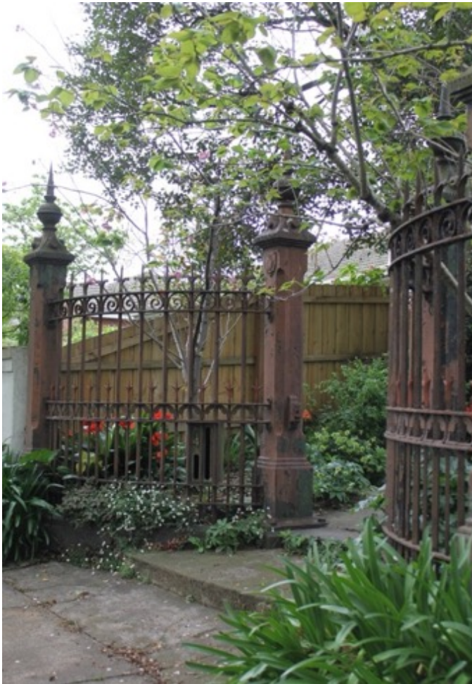
Figure 12 Cullymont – Subject Property Gate Entry – Gateway 1 – Palisade gate + fencing [cast-iron + wrought-iron] - Looking east [north-east] [left]
