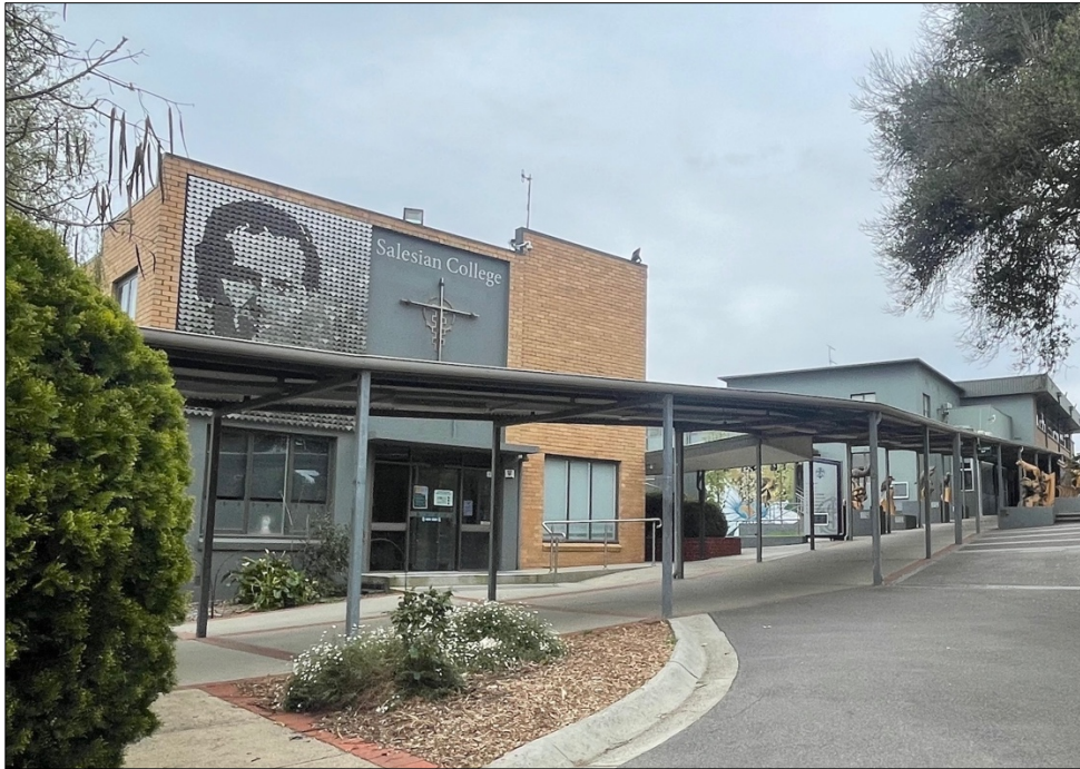
Figure 8 Post war/modern school buildings south-east of the chapel site.
