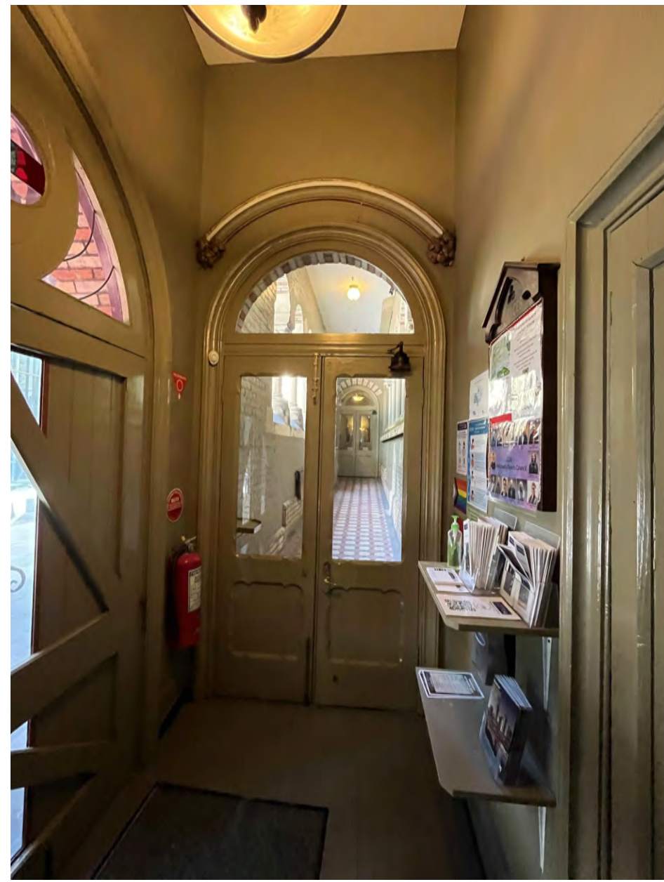
EXISTING - SITE PHOTO - EAST LOBBY LOOKING SOUTH
