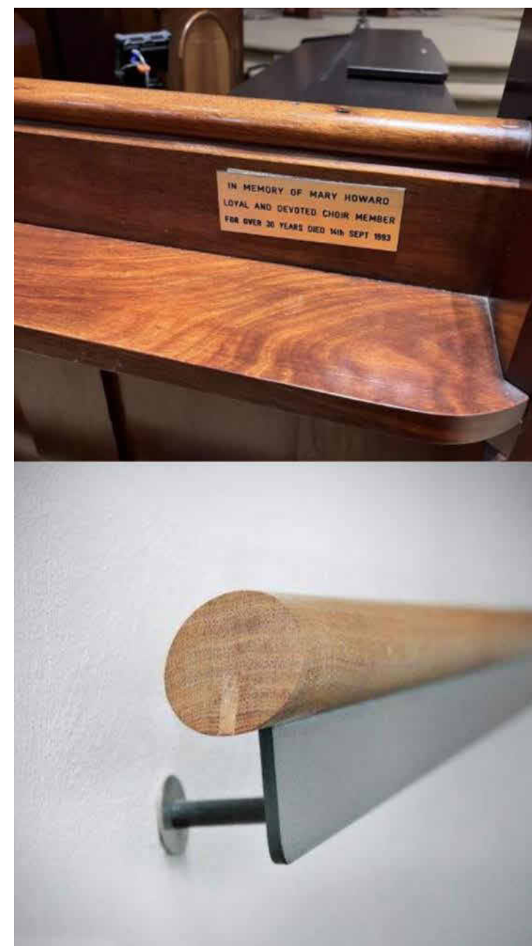
TM-03 TIMBER HANDRAIL FROM EXG PEWS
