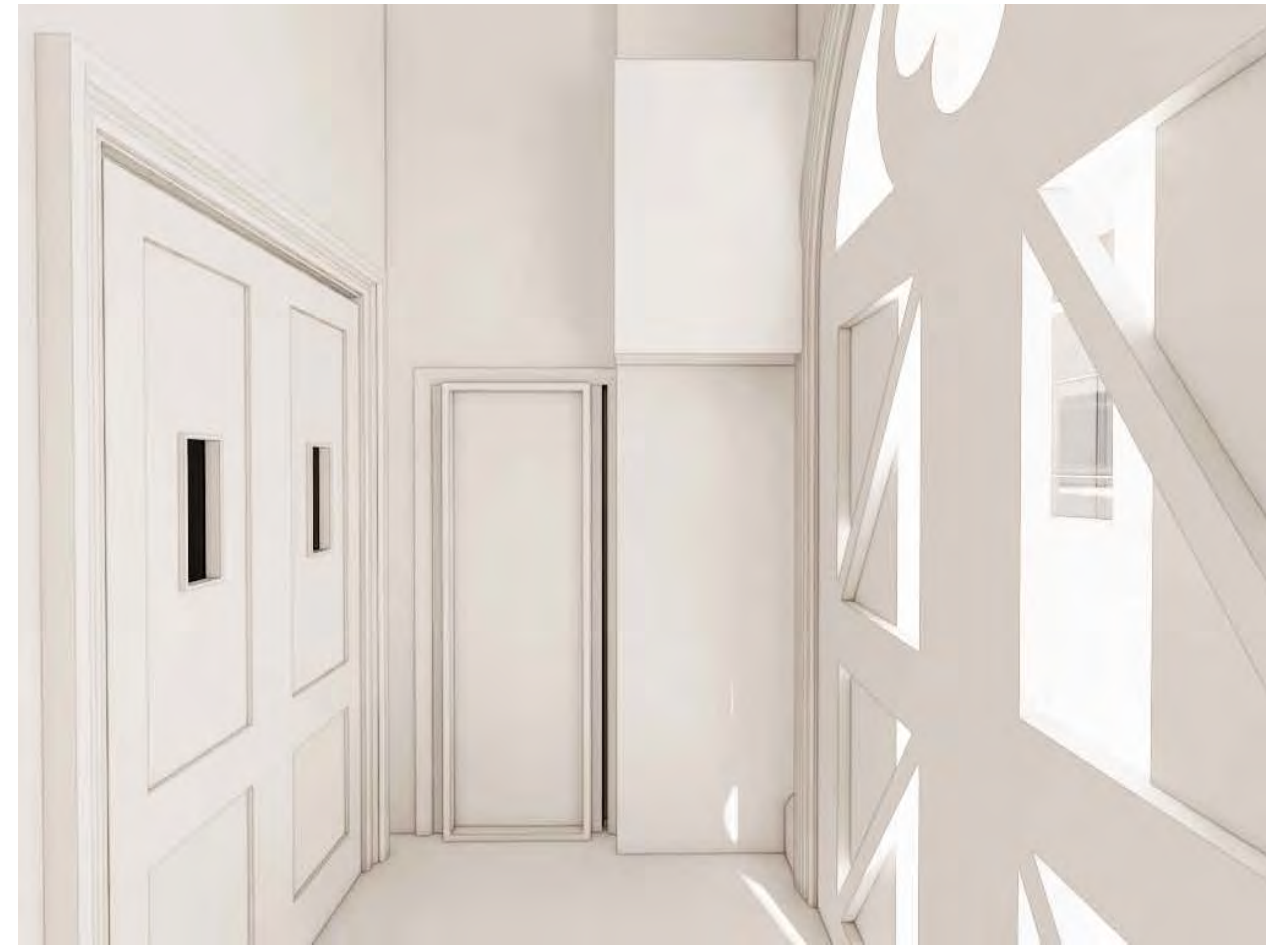
01. EXISTING - EAST LOBBY
