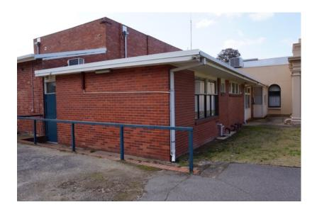
Figure 14: The north west (side) elevation of the Heathcote Civic Precinct viewed from within the site. The end of the original 1860s portion of the hall is indicated with an arrow, the remainder towards the rear was built in stages from the 1890s. Source of image: Peter Andrew Barrett Collection.
