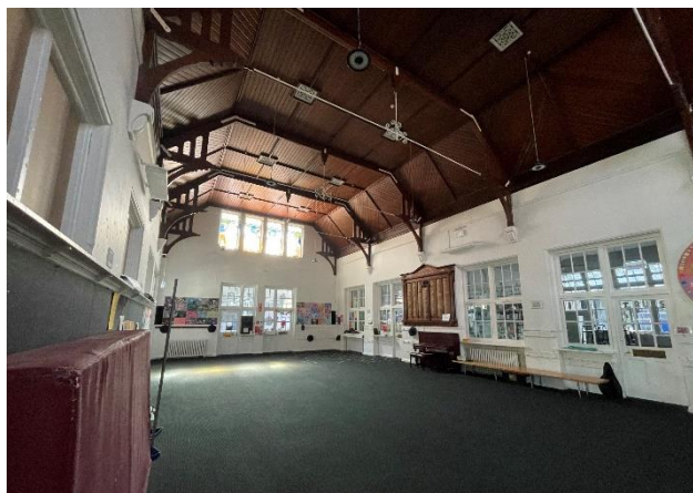
Figure 6 1914 building main hall (28/09/2023)
