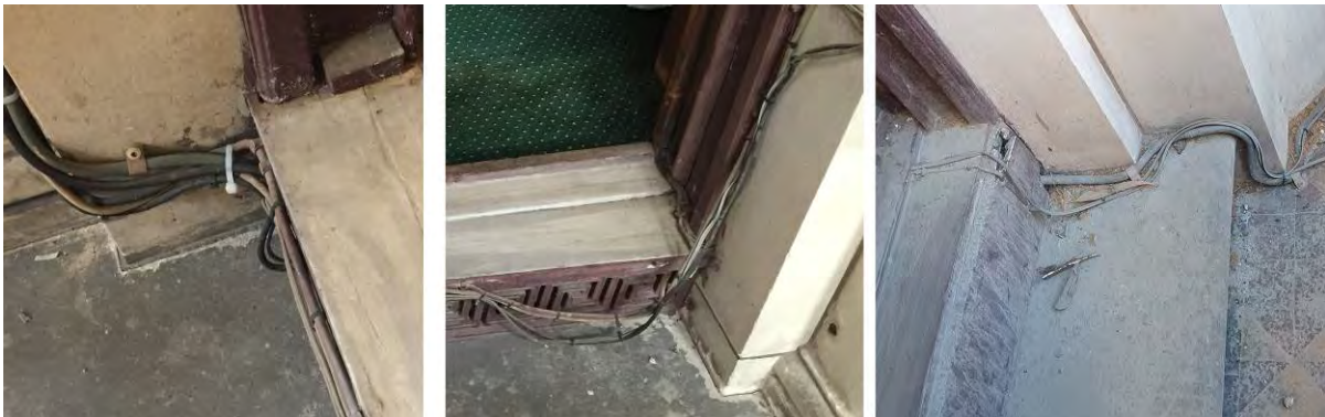
Images: Examples of previous cable penetrations which can cause and exacerbate damage (above), and examples of cabling reticulation in the past that can be visually disruptive and conspicuous (below)
