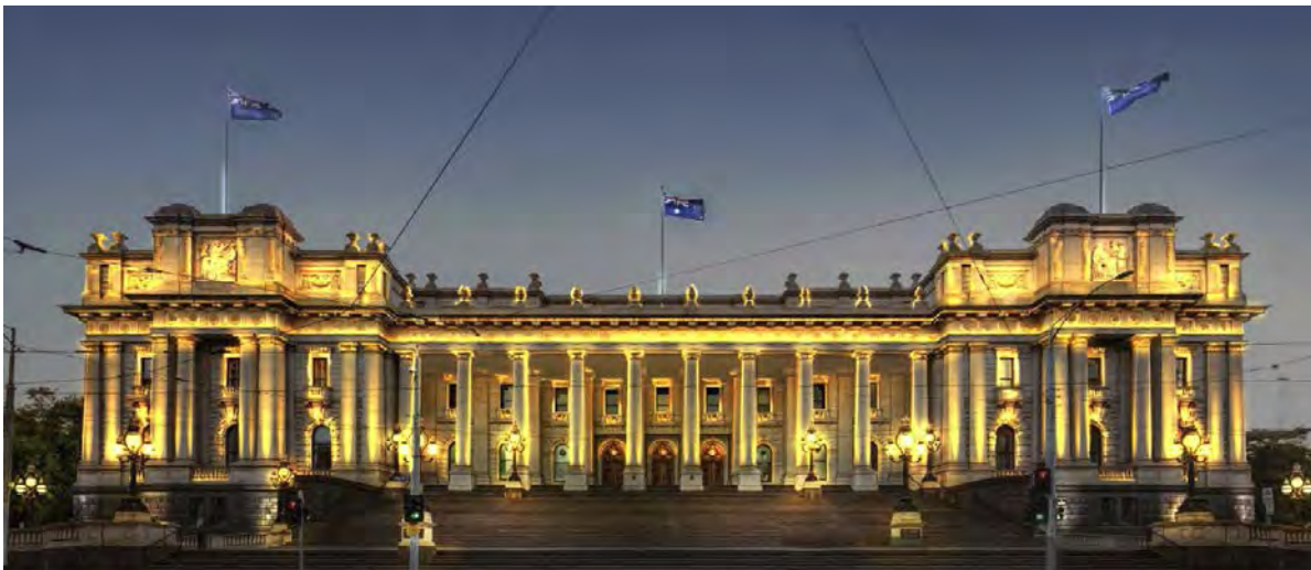
Images: Render produced by project Lighting Design Consultants F-POV to indicate project conceptual design intent only. Refer to F-POV presentation in Appendix.
