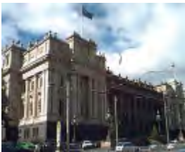
parliament house grounds works & fences spring street melbourne view from spring street
