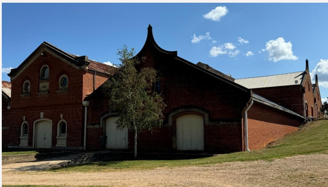
Figure 9 | North-east corner of building
