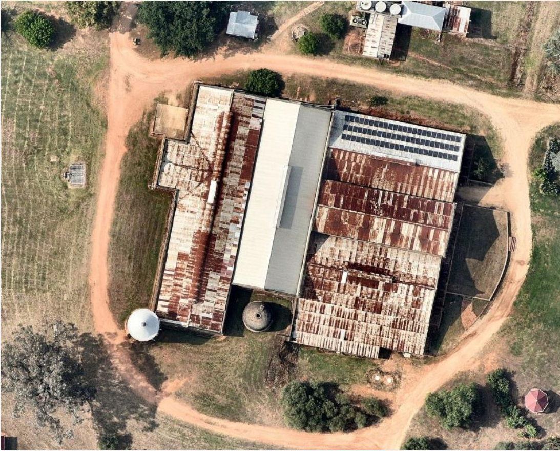
Figure 4 | Aerial view of development area (Source: Nearmap December 2023)
