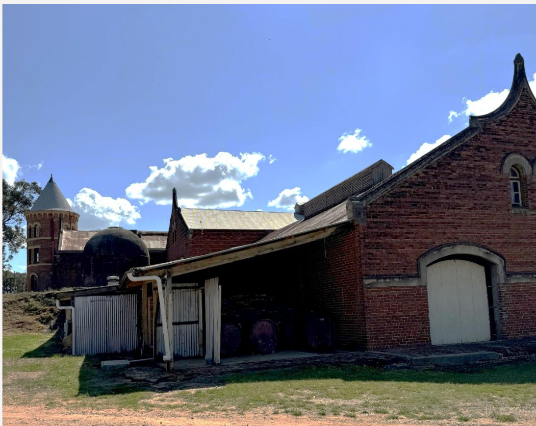
Figure 8 | South-east corner of building
