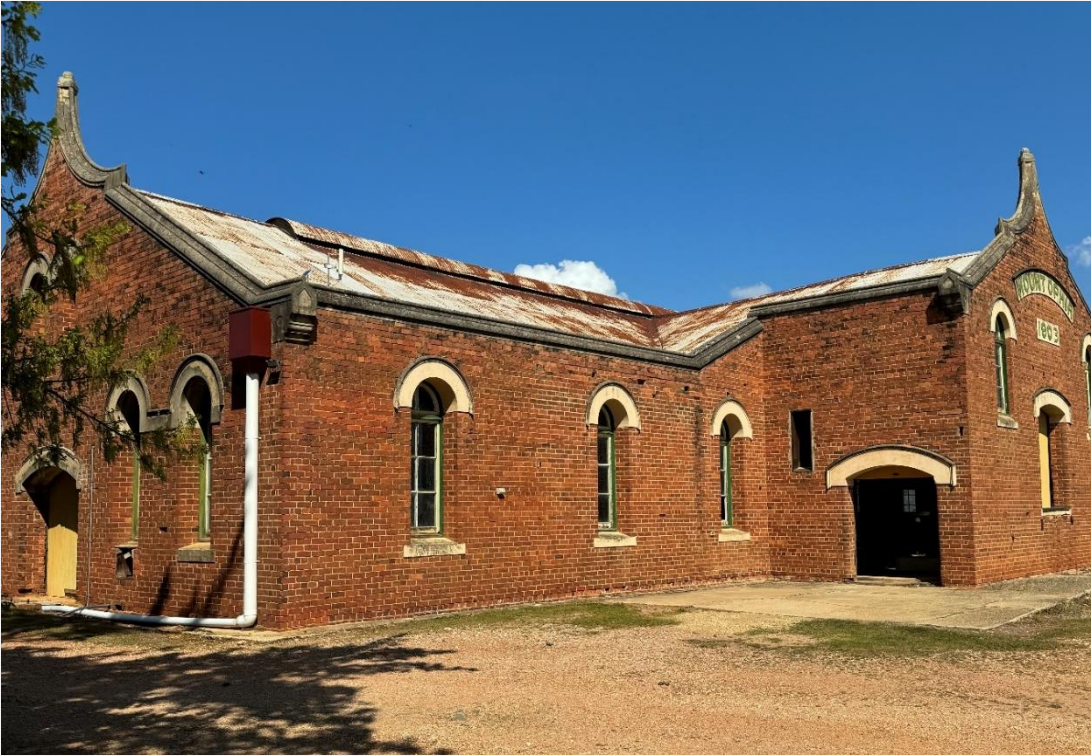
Figure 6 | North-east corner of building
