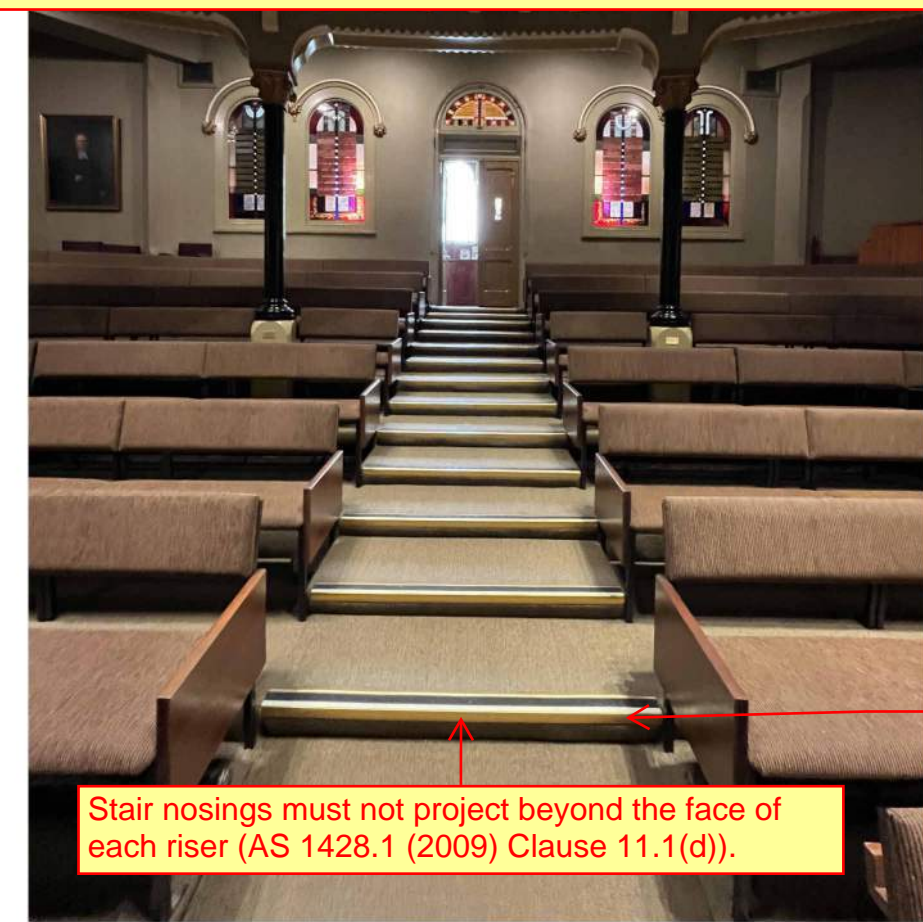
EXISTING UPPER STEPS
