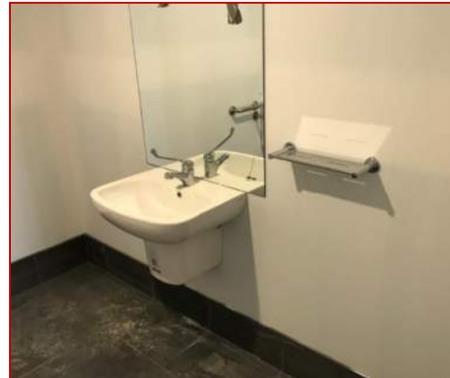
Example Compliant Accessible Washbasin
