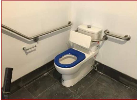
Example Compliant Accessible Toilet
