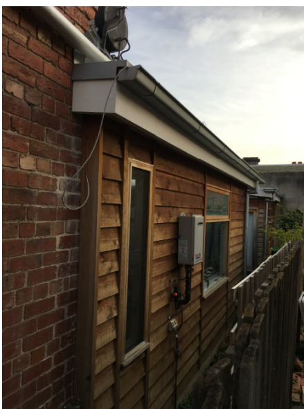
10. adjoining property - 116 Paterson Street view north
