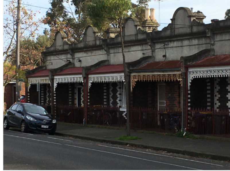
2. Paterson Street - street view
