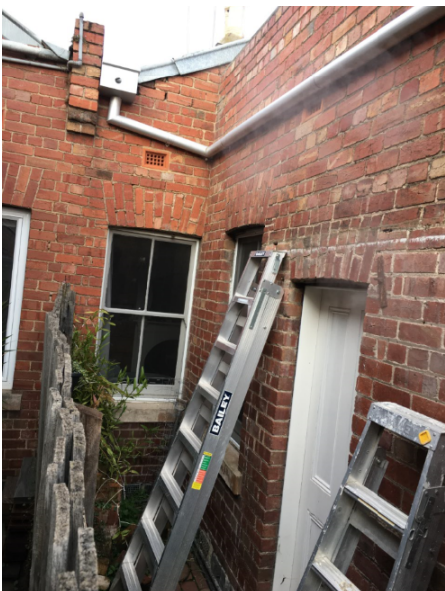
9. adjoining property - 116 Paterson Street lightwell
