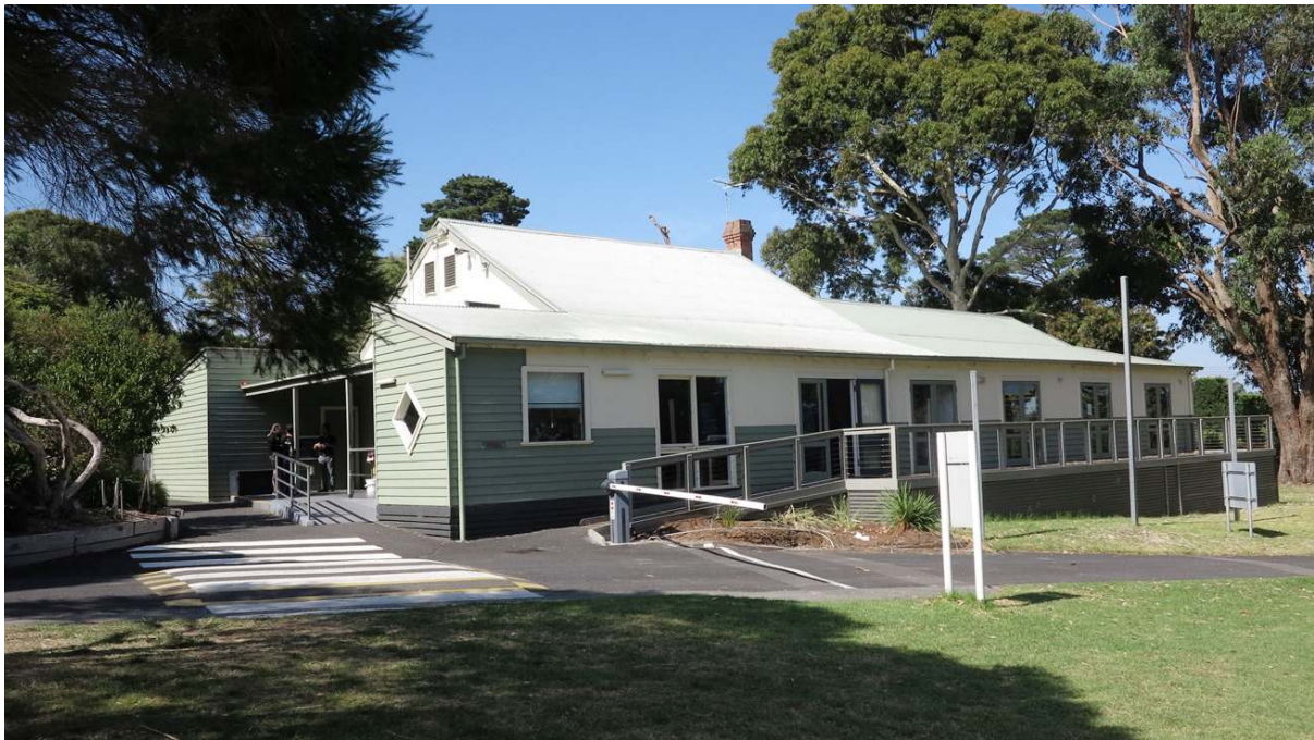
View from recreation area to northern roofs of the Hall Dining building (B1)
