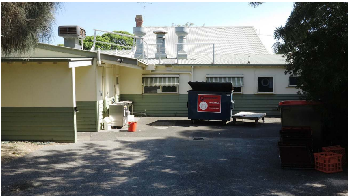
Southern side roofs of B1 showing existing kitchen vents in the 1990s extensions made to the building.
