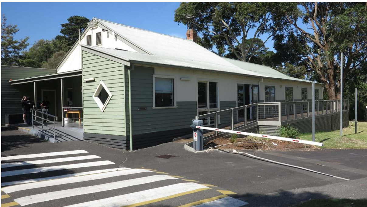
Close-up view from recreation area to northern roofs of the Hall Dining building (B1)
