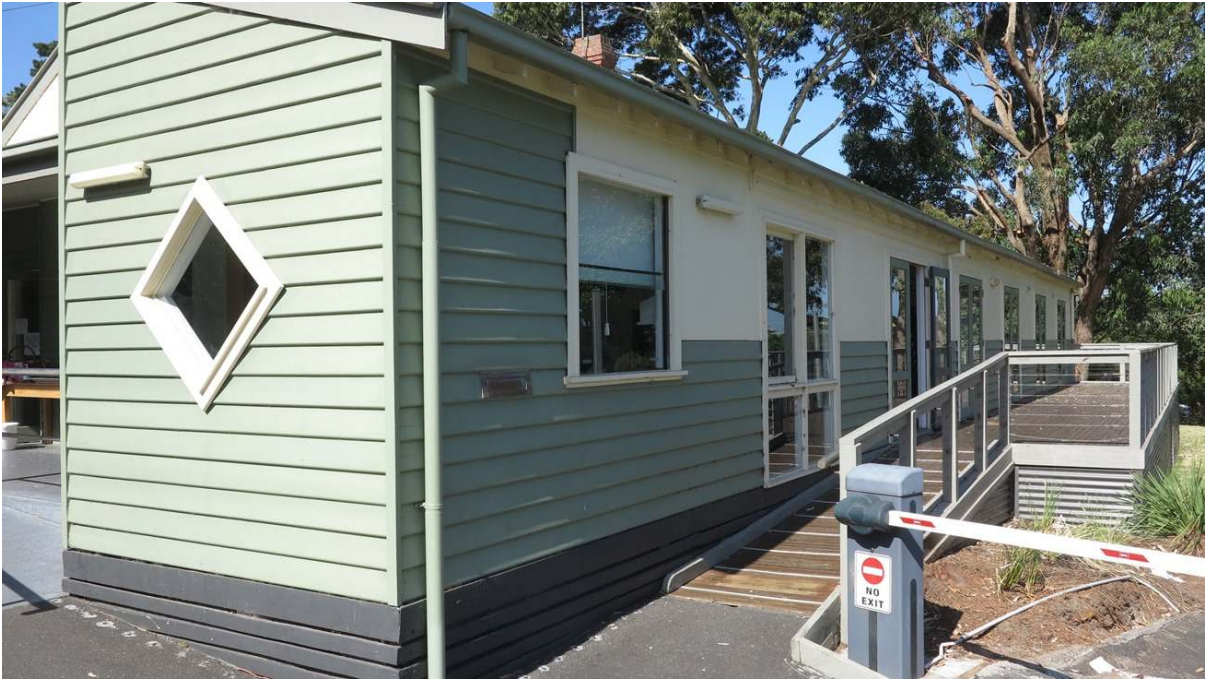
Verandah area to be placed under proposed shelter extension Building B1
