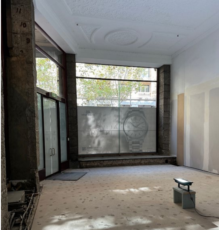
Figure 2 View of the interior ground floor of the tenancy
