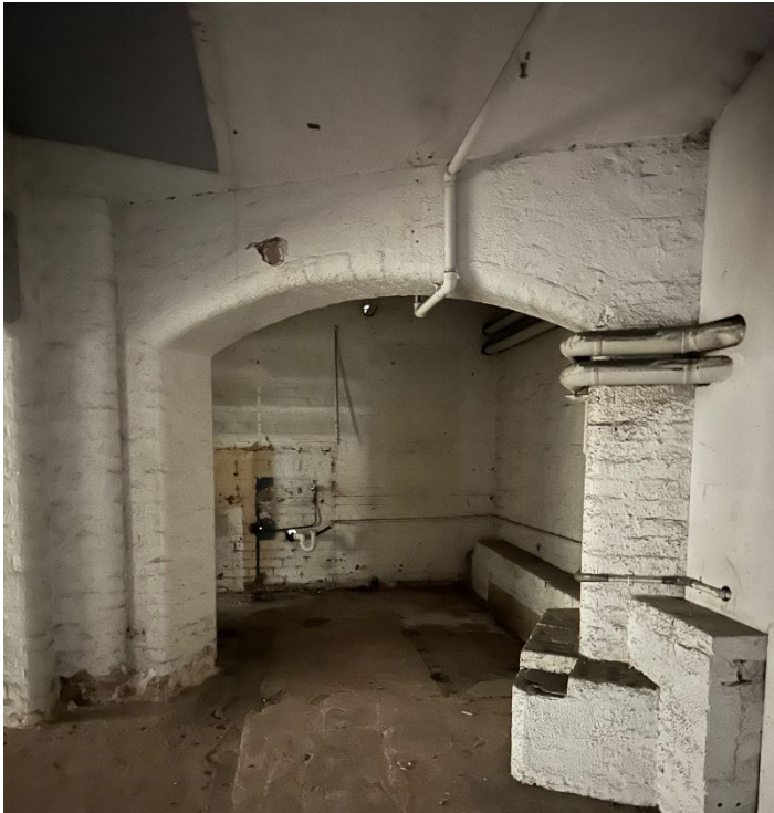
Figure 4 View of the basement space.
