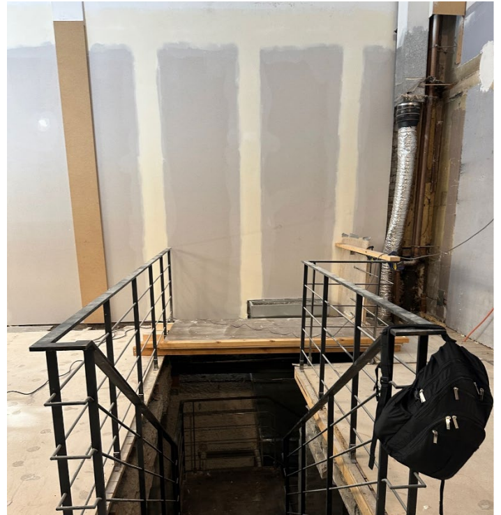
Figure 7 Existing stair within the tenancy space.
