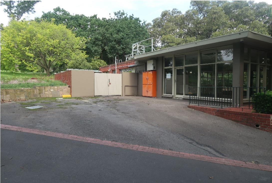
Figure 14 View from the west to the north façade with glazed addition
