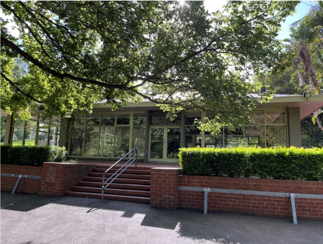
Figure 10 View from the west of the Pavilion's entrance stairs and terrace and the glazed façade set beneath the hipped slate roof
