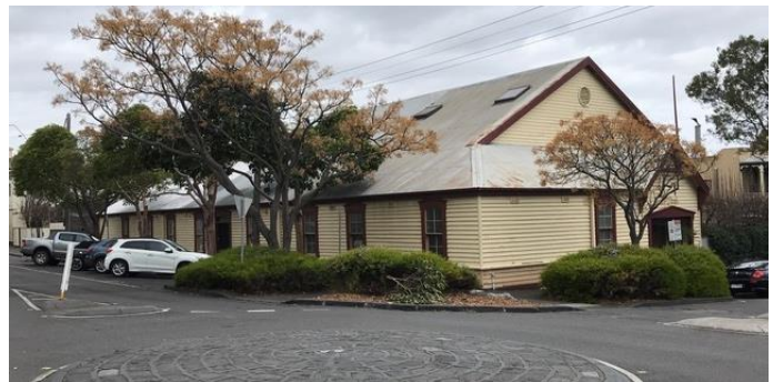
View from north east - eastern elevation (LHS) and west elevation (RHS) - showing lack of roof spaces due to gable end configuration of the rectangular roof aligned east west and facing north.
