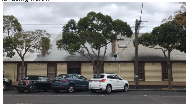
LHS south elevation - note cut out sections of roof for outdoor courtyards and therefore limited roof slope on this elevation, in addition, a south facing roof is the least satisfactory location for solar panels.
