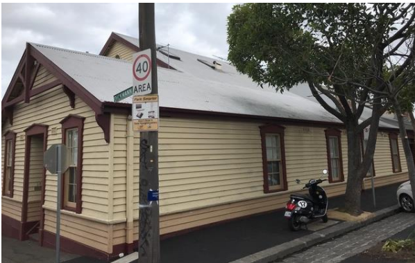
View from north east - eastern elevation (LHS) and west elevation (RHS) - showing lack of roof spaces due to gable end configuration of the rectangular roof aligned east west and facing north.
