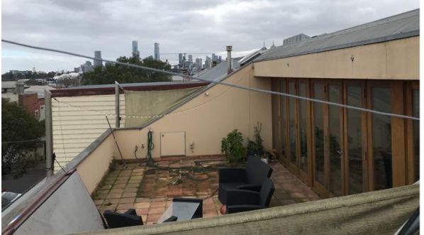
LHS south elevation - note cut out sections of roof for outdoor courtyards and therefore limited roof slope on this elevation, in addition, a south facing roof is the least satisfactory location for solar panels.
