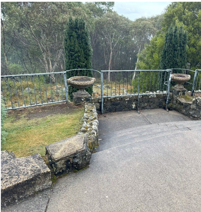
Figure 15 Existing safety railing from podium interior, showing existing alignment around urns.
