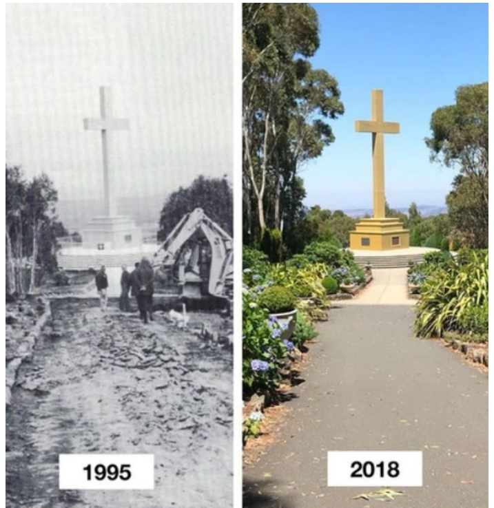
Figure 10 The site 1995 during major works in comparison to 2018. Source: Mount Macedon ANZAC Day Dawn Service.
