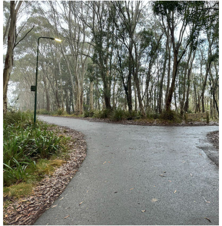
Figure 14 Existing Mount Macedon Memorial Cross Walk pathway lighting.
