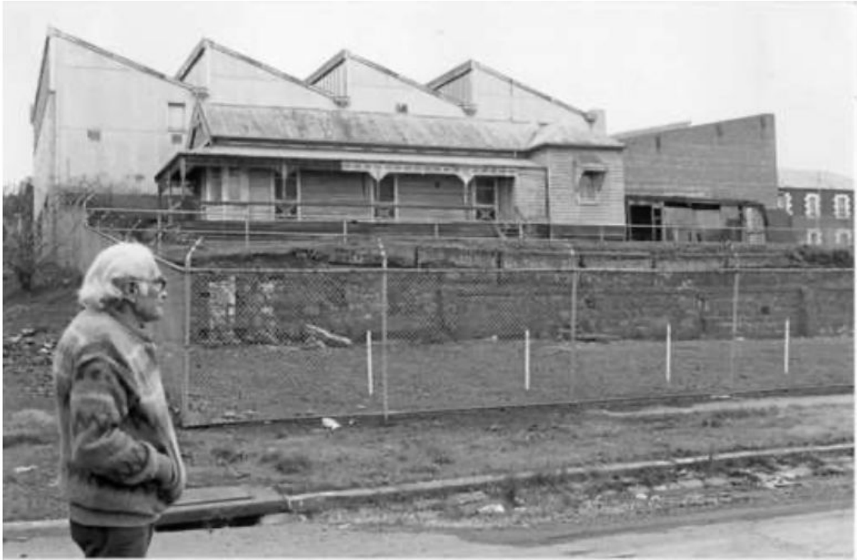
Figure 2: Excerpt from Biosis Report : Demolished Ship Inn, Maribyrnong Street 1980 (Footscray Historical Society) note the surviving rear bluestone retaining wall
