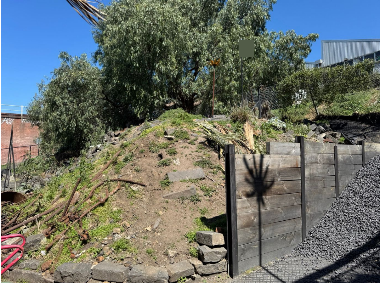
Figure 6: Photograph of the fill and rubble, and large peppercorn tree (view from Waterside Metal Art site)
