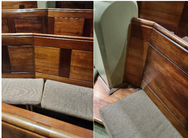
Figure 15 Choir stalls in their current curved arrangement. Note: physical evidence of altered/joined panels. Source: Trethowan Architecture, 2024.
