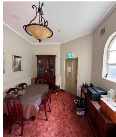
Figure 34 Choir Vestry. Note painted rendered plinth to LHS of image. Source: Trethowan Architecture, 2024.
