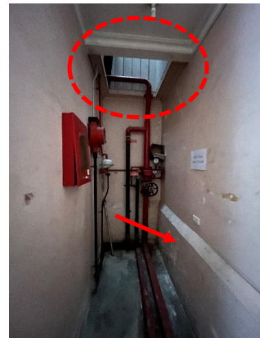
Figure 37 Fire Services Room looking south. Note skylight (indicated by red circle) and plinth to original west wall of church (indicated by red arrow). Source: Trethowan Architecture, 2024.
