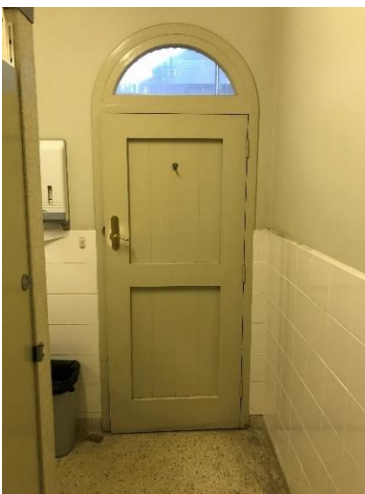
Figure 31 Toilet facilities looking east to external door. Source: Trethowan Architecture, 2024
