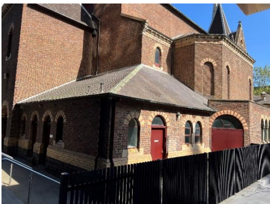
Figure 21 Single-storey amenities addition to the north-east corner as viewed from St. Michael's Walk. Source: Trethowan Architecture, 2024.
