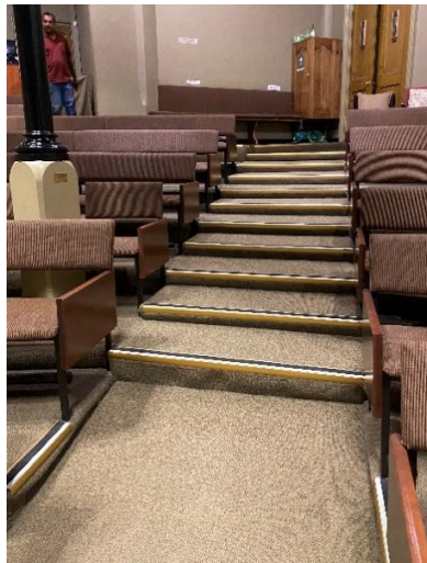
Figure 28 Tiered seating looking towards the rear of the Auditorium. Source: Trethowan Architecture, 2024.
