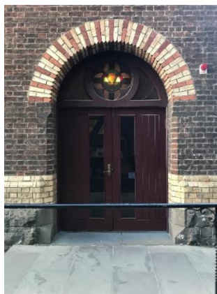
Figure 22 St. Michael's Walk entrance doors. Note, later glazed panels. Source: Trethowan Architecture, 2024.
