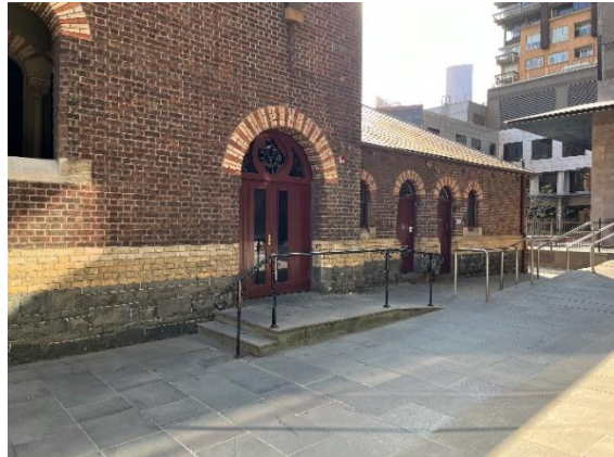
Figure 18 Accessible entrance to St. Michael's Walk. Source: Trethowan Architecture, 2024.
