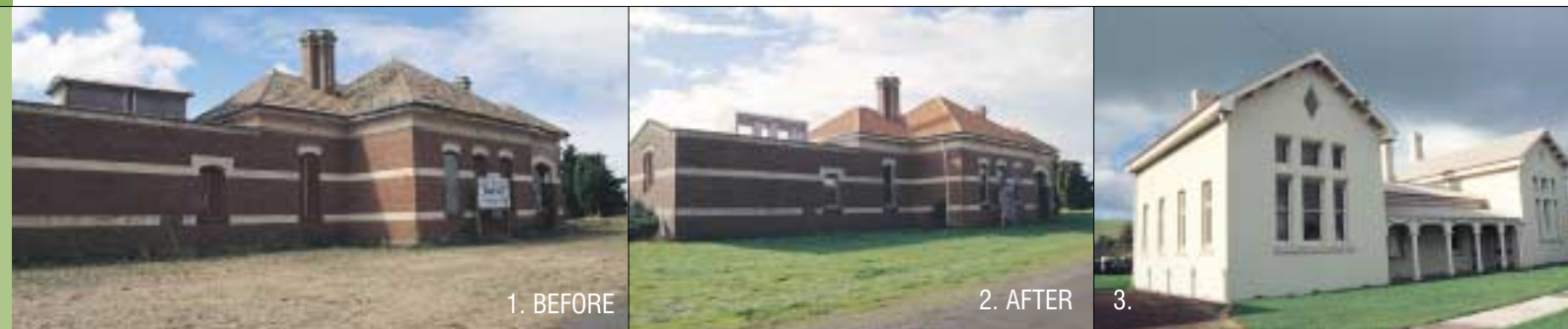
1. BEFORE - KOROIT RAILWAY STATION IN A VERY POOR STATE 2. AFTER - KOROIT RAILWAY STATION CAN BE USED ONCE AGAIN 3. FORMER WANNON SHIRE OFFICES, COLERAINE
