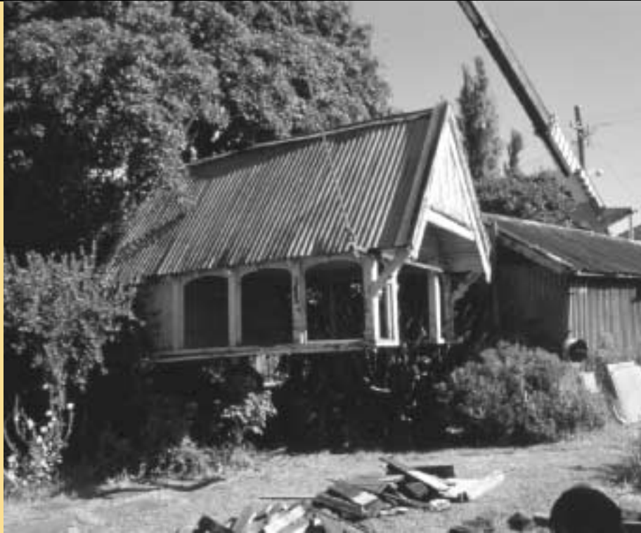
Removing the shelter from South Yarra
