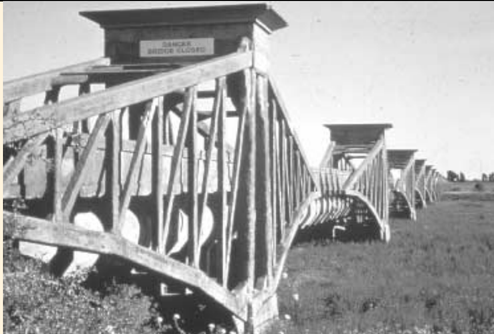
Ovoid Sewer Aqueduct, Geelong
